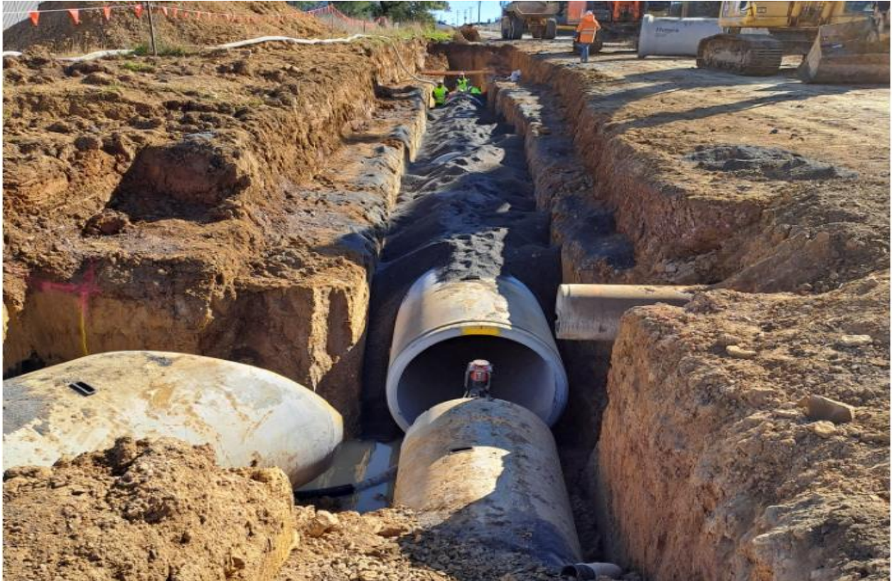
Photo – Precast concrete drainage pipes being laid on Clergate Road
