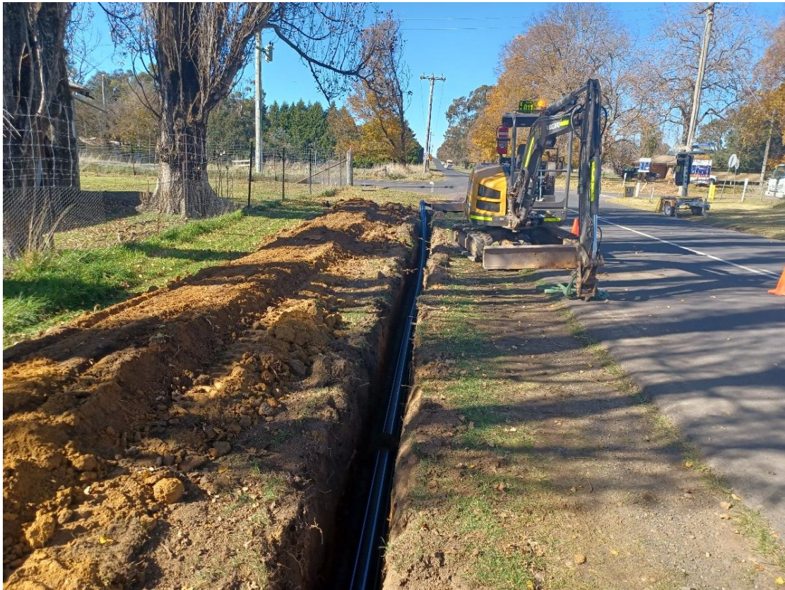
Photo – Trenching and Pipe Laying – Water Main – Canobolas Road
