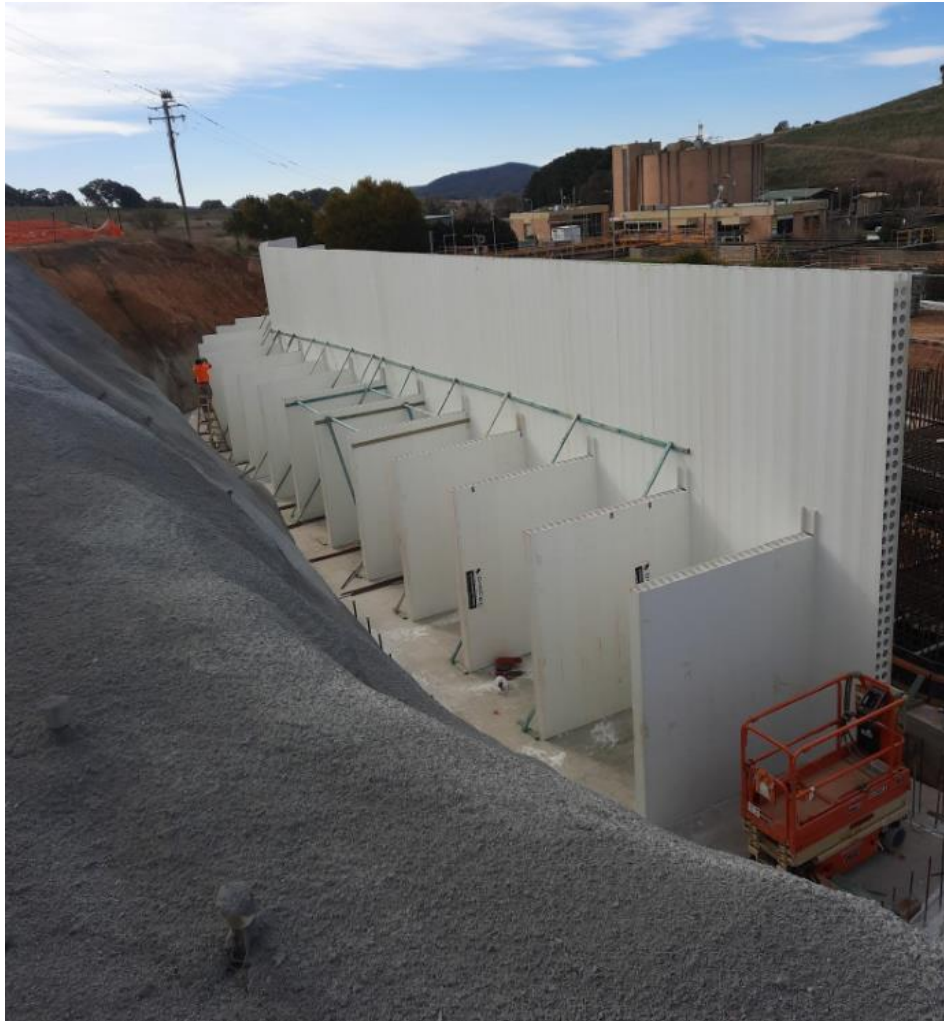
Photo – STP Inlet Works – retaining wall
