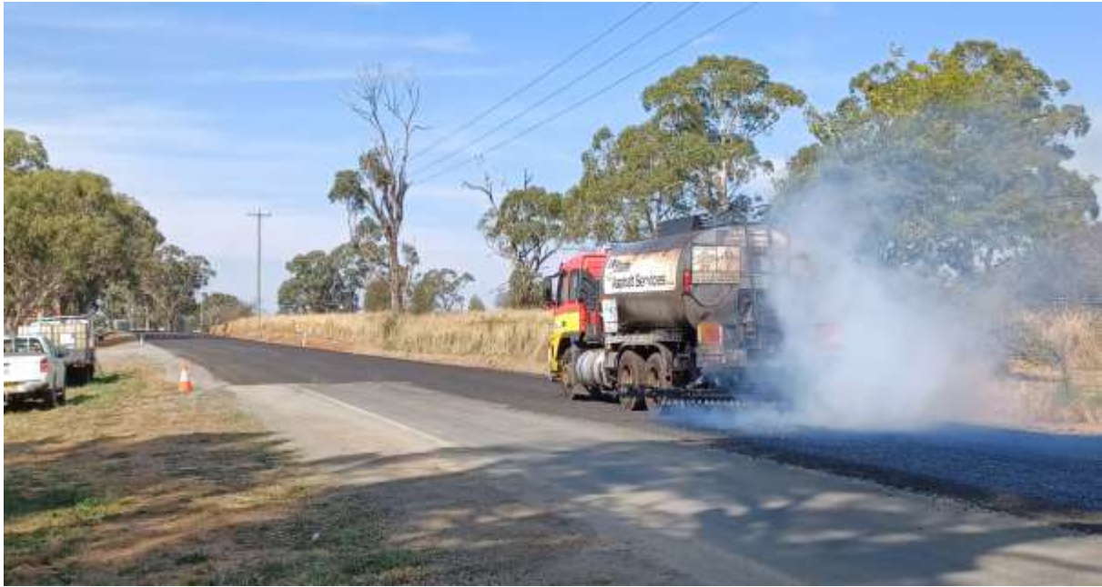
Photo – Sealing new works on Forest Road
