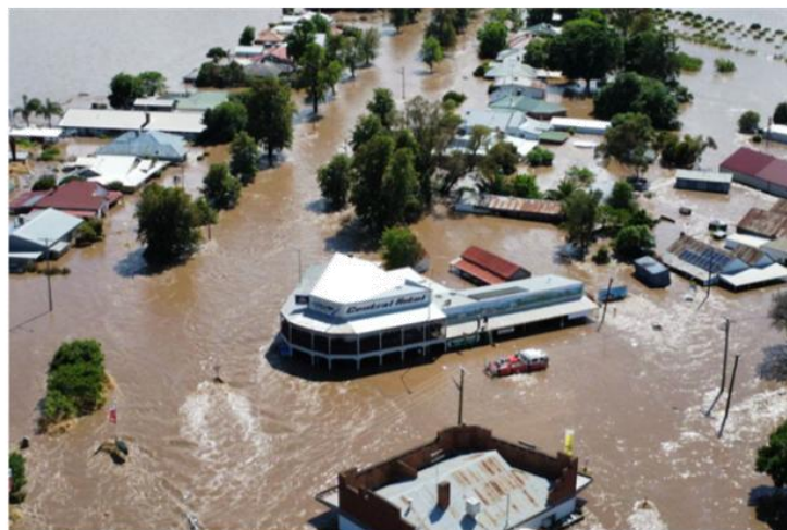
Figure 5: Recent floods devastated regional towns, including Eugowra in November 2022, where two lives were lost, and key infrastructure like Nyrang Bridge was severely damaged. Road damage hindered response efforts, highlighting the urgent need for funding models that prioritise community resilience.
