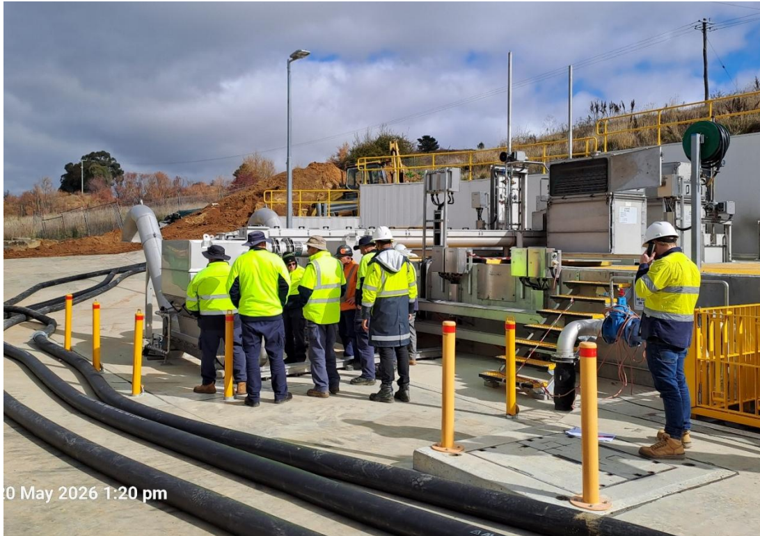
Photo – STP Inlet Works – training in progress
