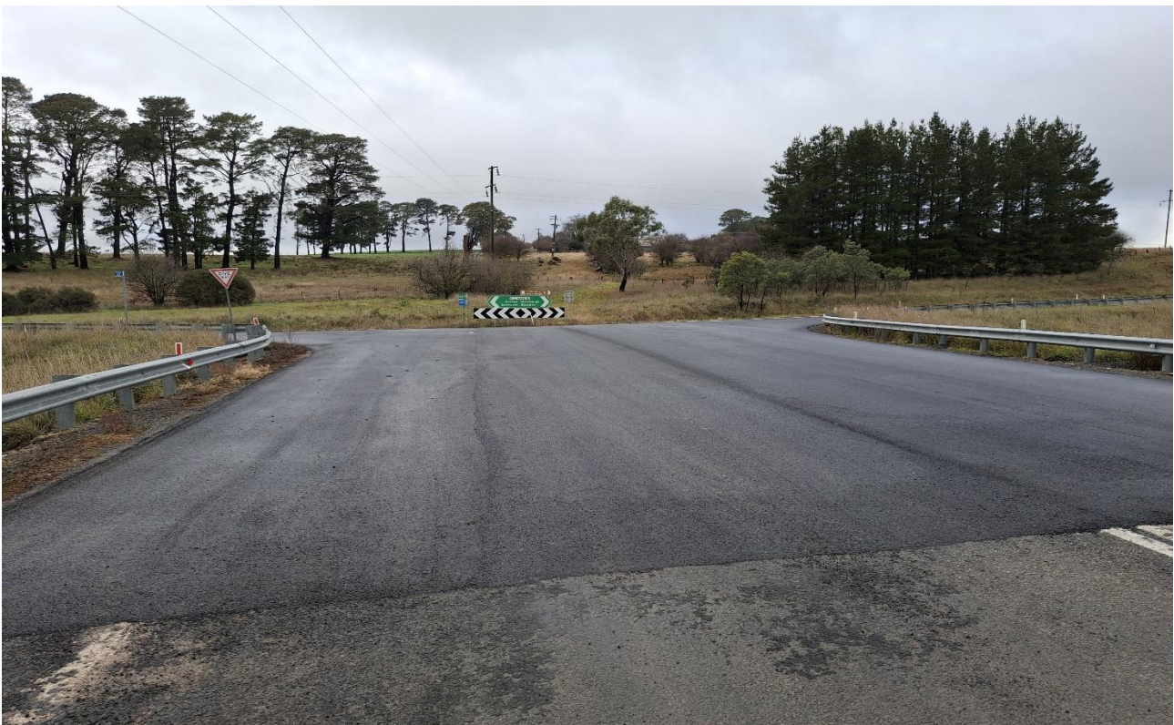
Photo: Asphalt tie in at Whiley Road and Millthorpe Road intersection
