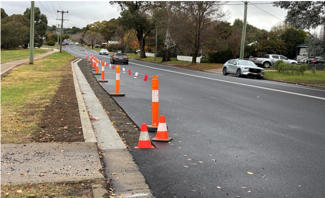
Photo: Kerb and gutter reconstruction on Woodward Street
