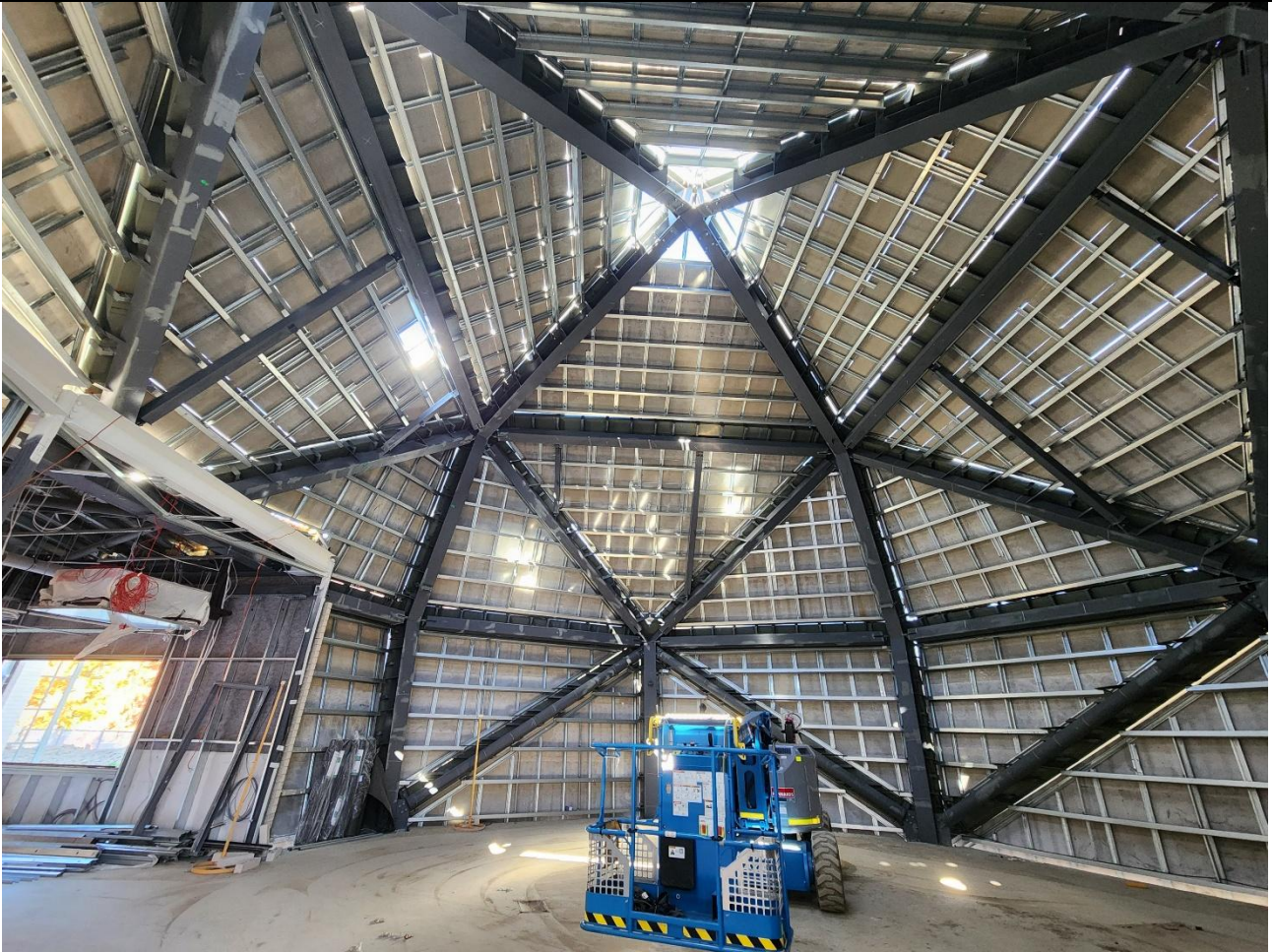
Photo – Construction of Orange Conservatorium and Planetarium – Dome Construction
