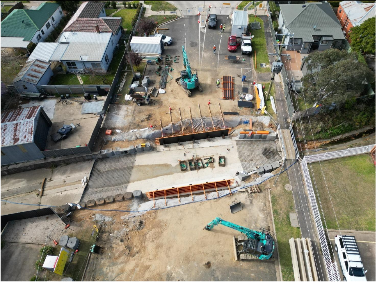
Photo – March Street Bridge – Floor slab of the channel being prepared.
