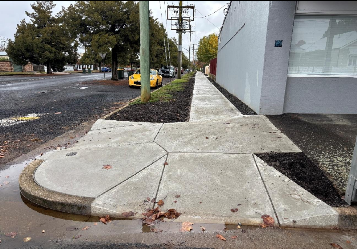
Photo: Footpath renewal on Clinton Street
