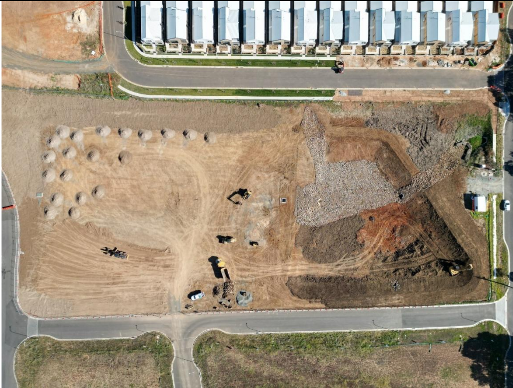
Photo – C2 Basin - Main field and basin being constructed
