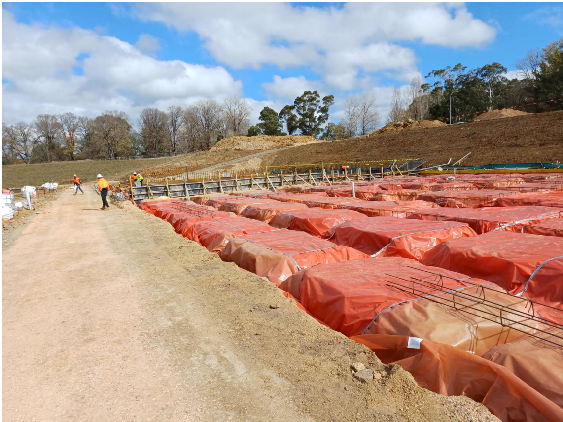
Photo – Sports Precinct – Main slab to JD Stadium being prepared
