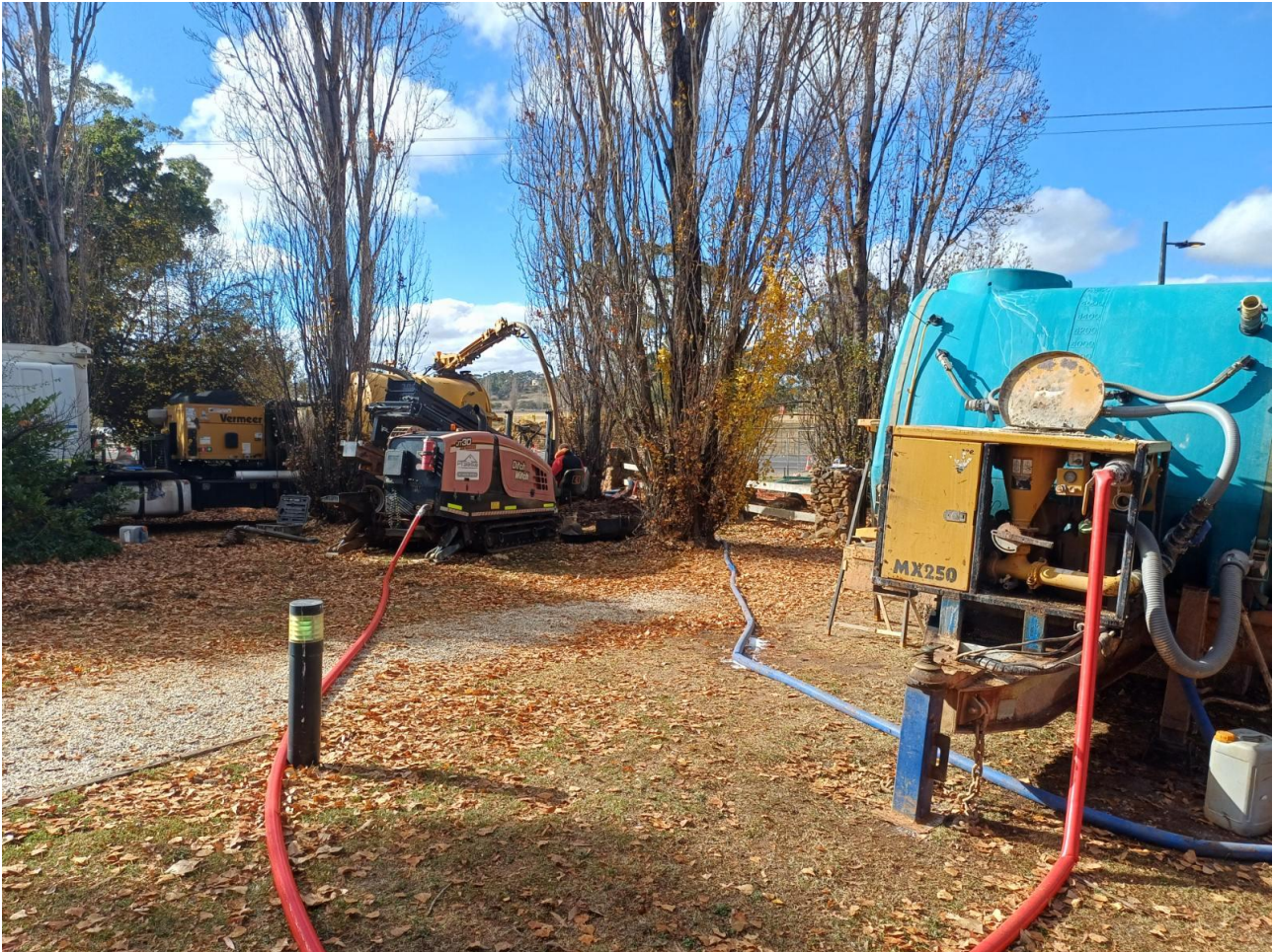
Photo – Sports Precinct – Electrical under bore of Forest Rd
