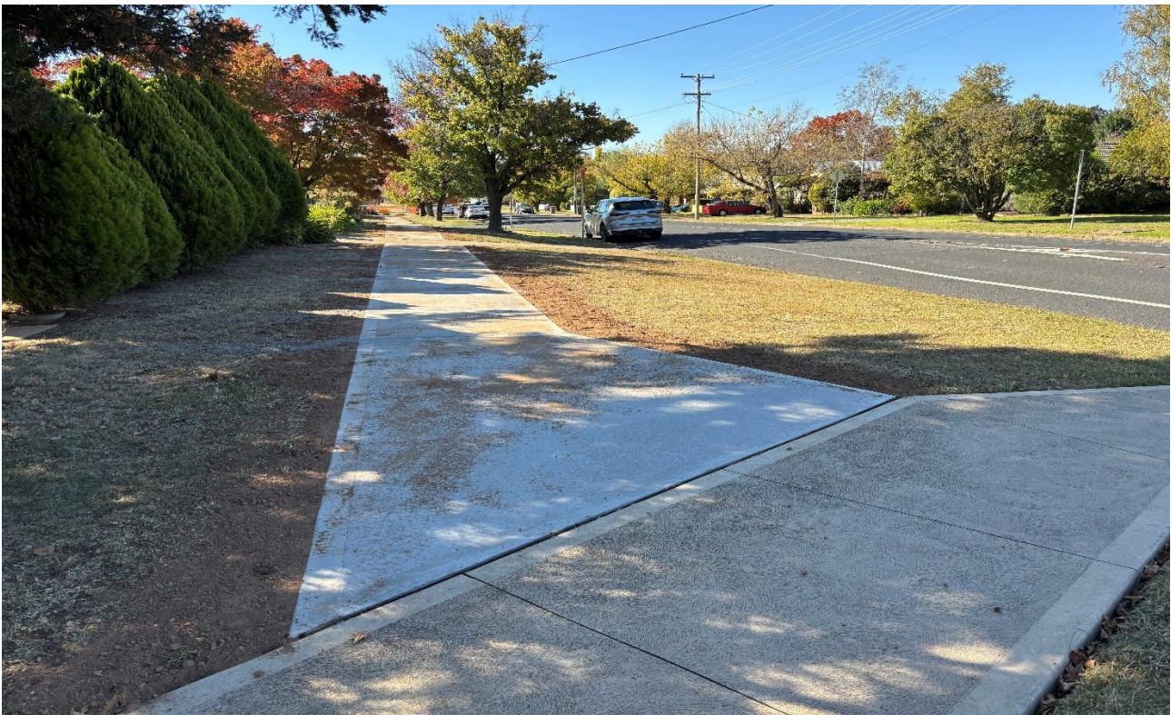
Photo: New footpath construction in Sampson Street
