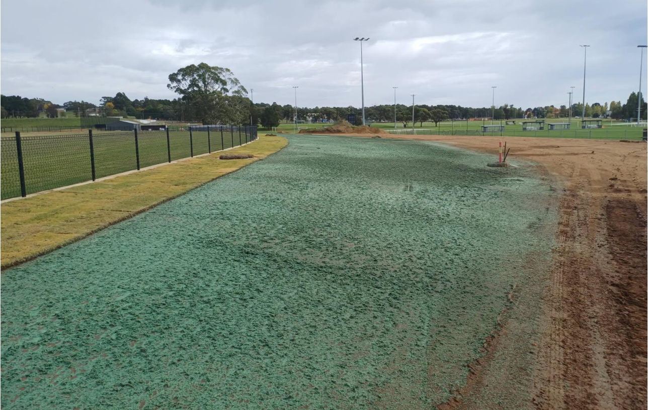
Photo – Sports Precinct - Landscaping and turfing of exterior fields 1-8
