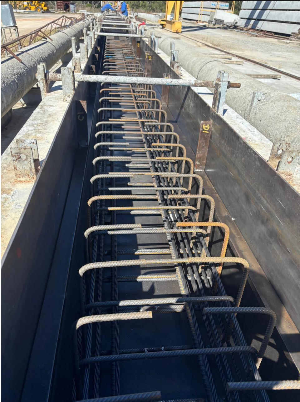
Photo – March Street Bridge - Precast beams being prepared off-site
