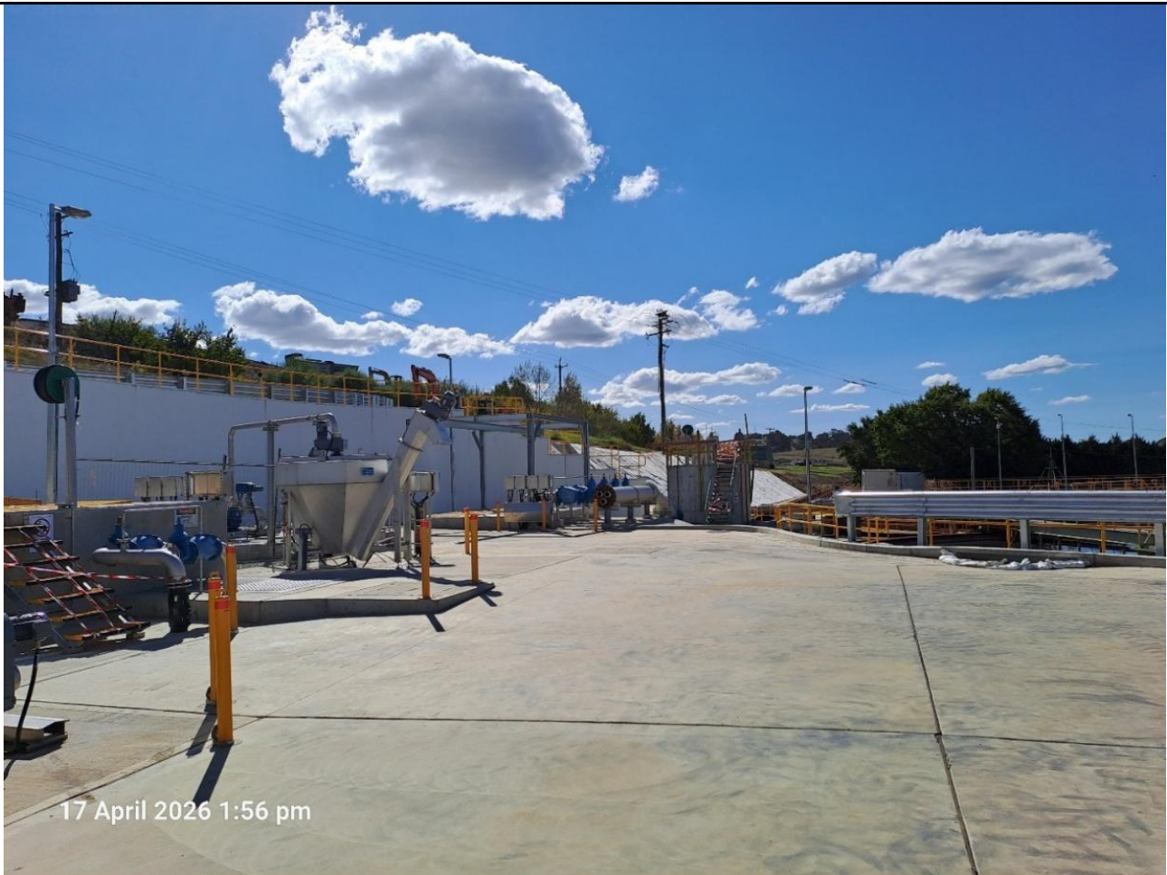
Photo – STP Inlet Works
