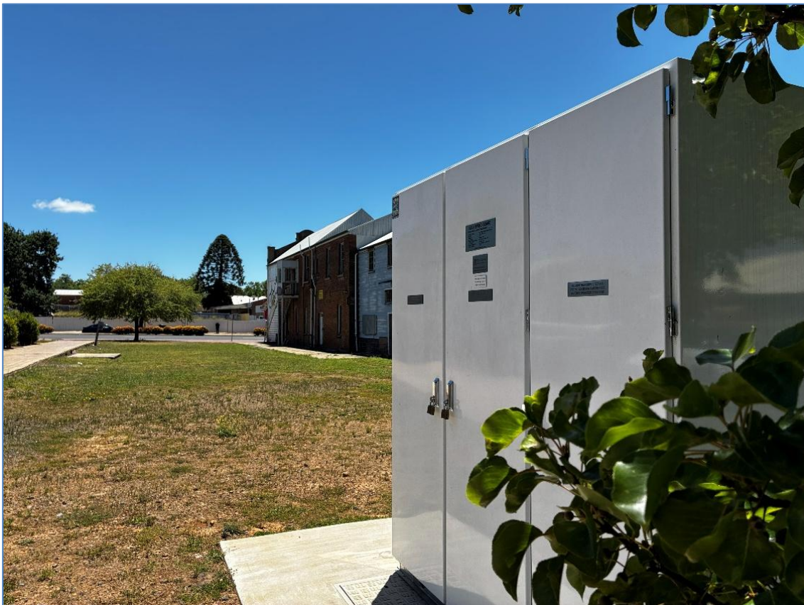
Figure 22 - subject site looking north, existing EV battery/substation adjacent to pedestrian path
