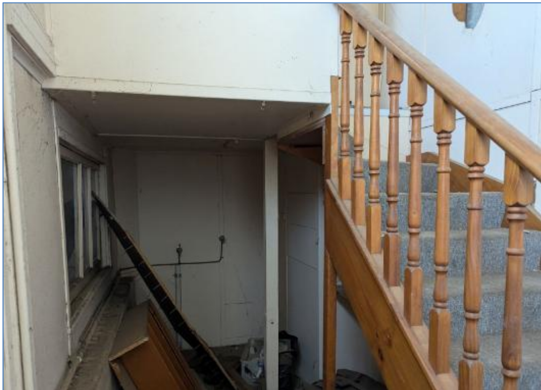
Figure 37 – modern refit staircase and fibre cement sheet partitions
