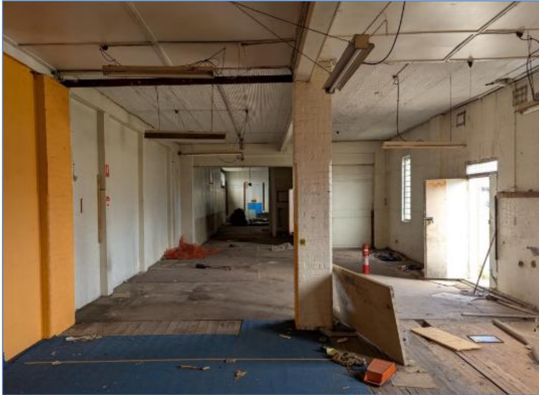
Figure 36 – backroom to the original building showing the transition between the shopfront and manufacturing floor. Note the transition of timber floorboard to concrete
