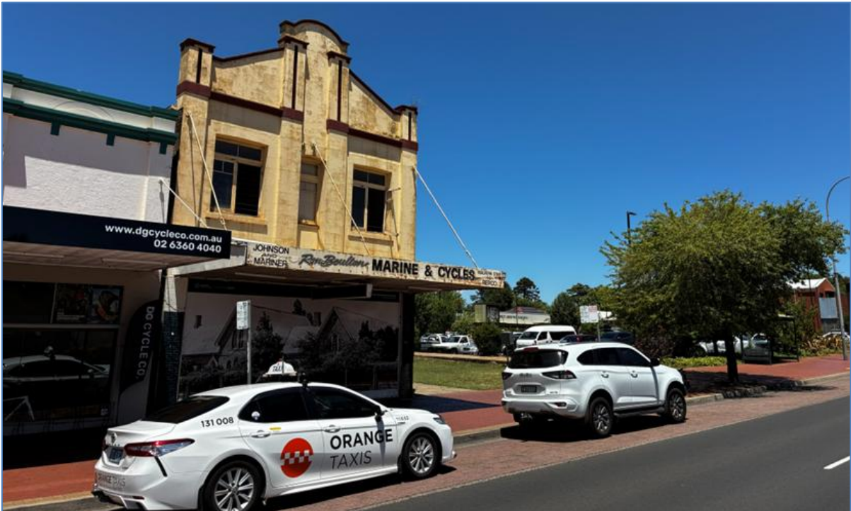
Figure 15a - 108 Summer Street building façade, awning and existing street tree Manchurian pear
