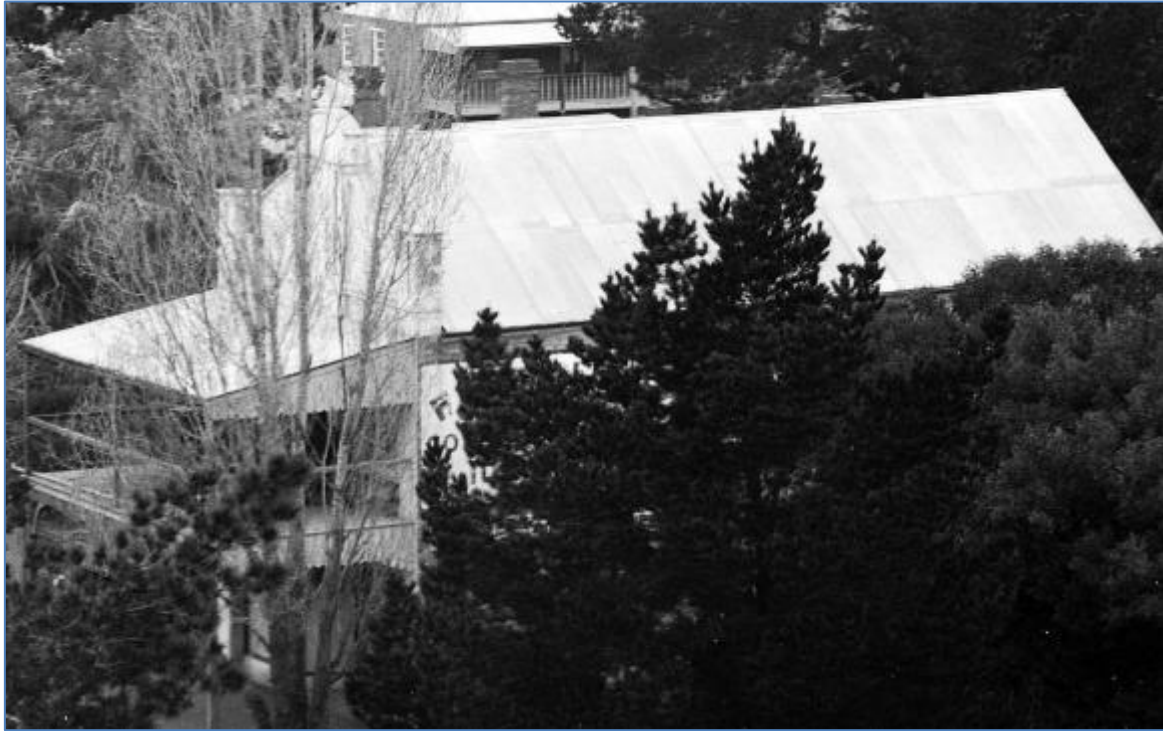
Figure 30 – photograph of the commercial building at 108 Summer Street c1920s viewed from the fire station tower (Source: O&DHS)
