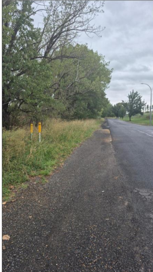
Figure 30: site inspection photo: - extent of pavement on Perc Griffith Way
