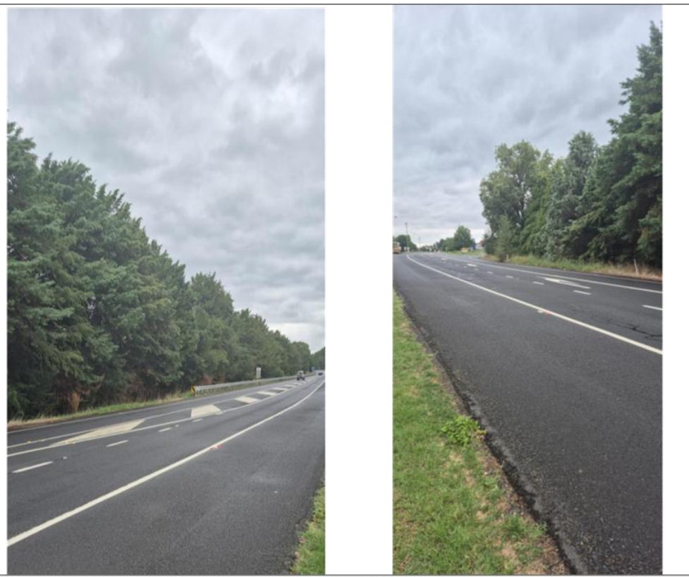
Figure 25: site inspection photos - Mitchell Highway (south-east)
