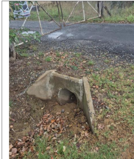
Figure 31: site inspection photo – existing vehicle access crossing
