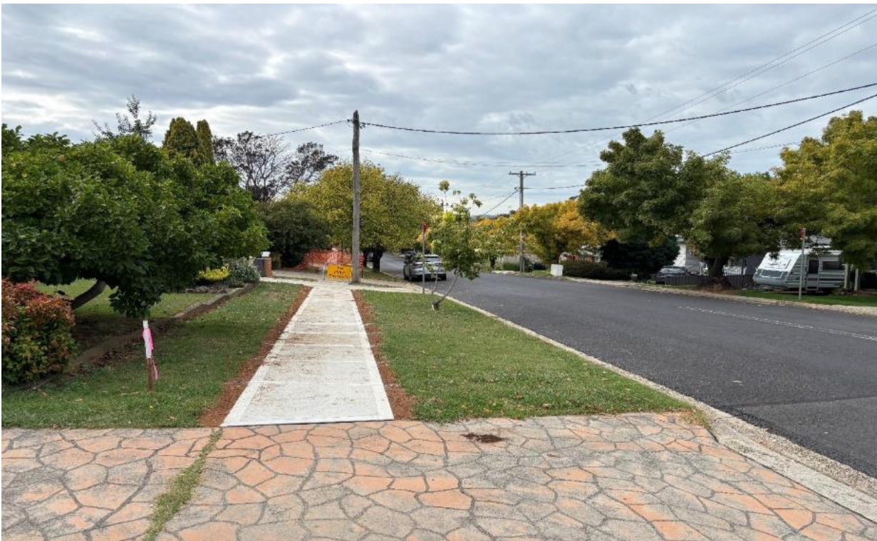
Photo: New footpath construction in Phillip Street
