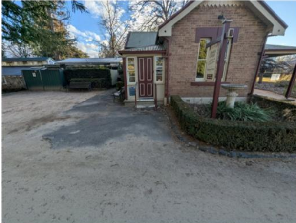
2. Entry view of front elevation
