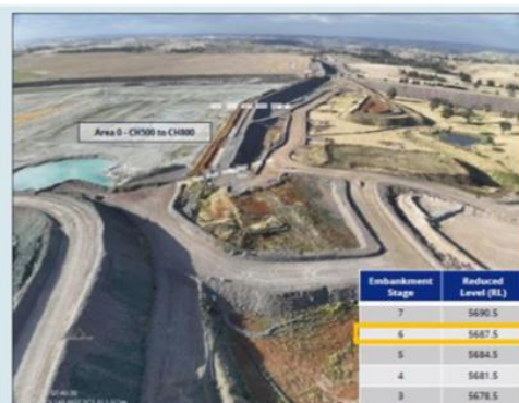
Image 4. STSF7 Western Embankment – Area 0 (January 2026)
