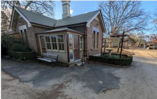
1. General view of the entry which is via the enclosed verandah
