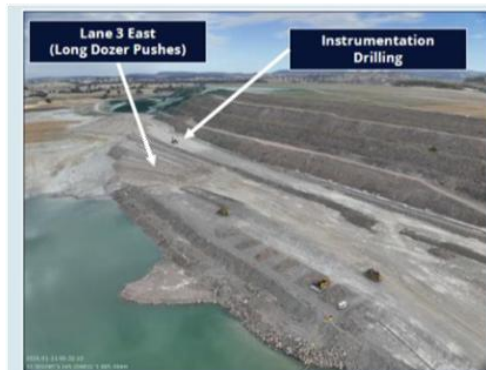
Image 3. NTSF Area 3 East Buttressing (January 2026)
