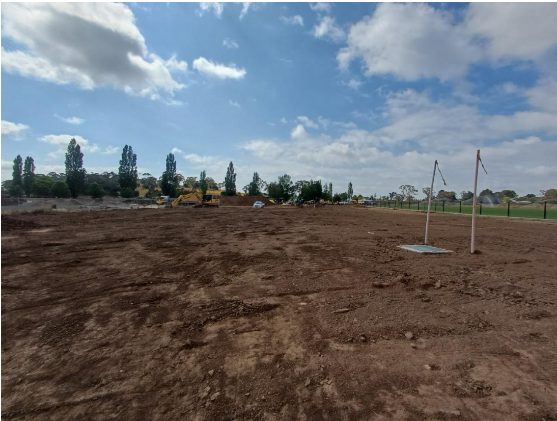
Photo – Sports Precinct – Spreading of Topsoil to Northern End of fields 1-8
