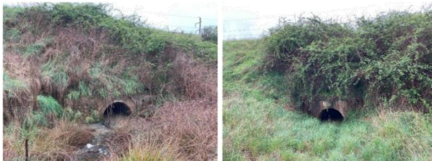
Figure 2-3: Blockage at the railway culverts (15 October 2025)
