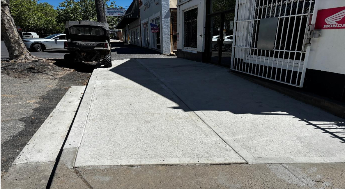
Photo – Footpath and gutter reconstruction outside of Morris Motorcycles
