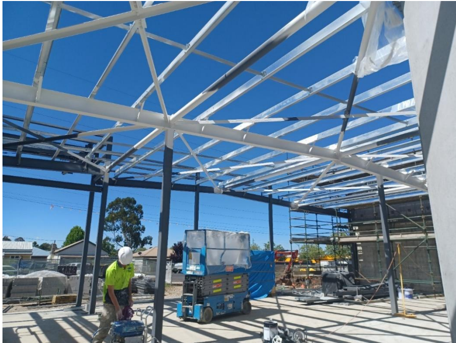
Photo – Construction of Orange Conservatorium and Planetarium – Back of house steel and intumescent painting installation underway.
