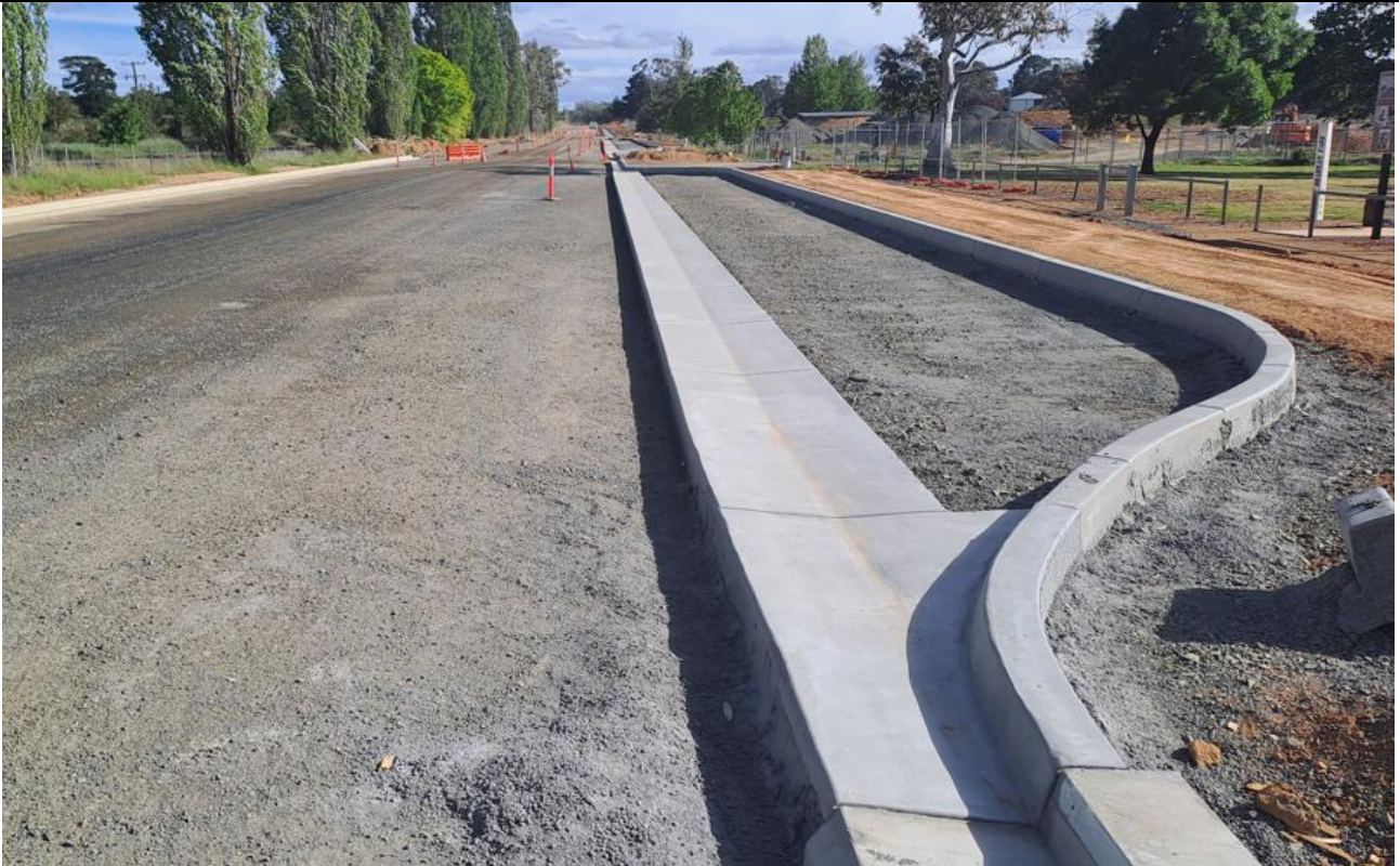
Photo – Huntley Road new kerb work for on street parking
