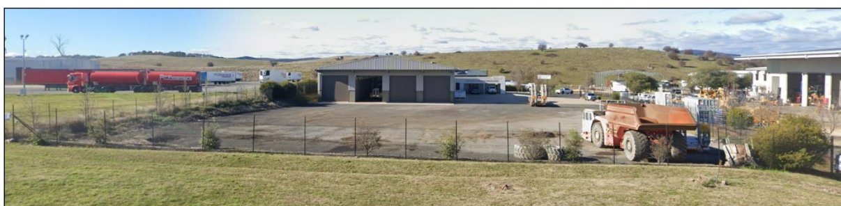
Figure 6 - existing street view from Northern Distributor Road
