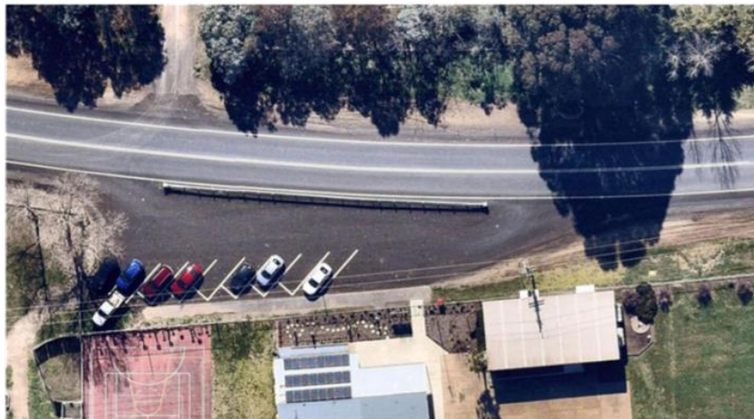
Photo: Post works completed
