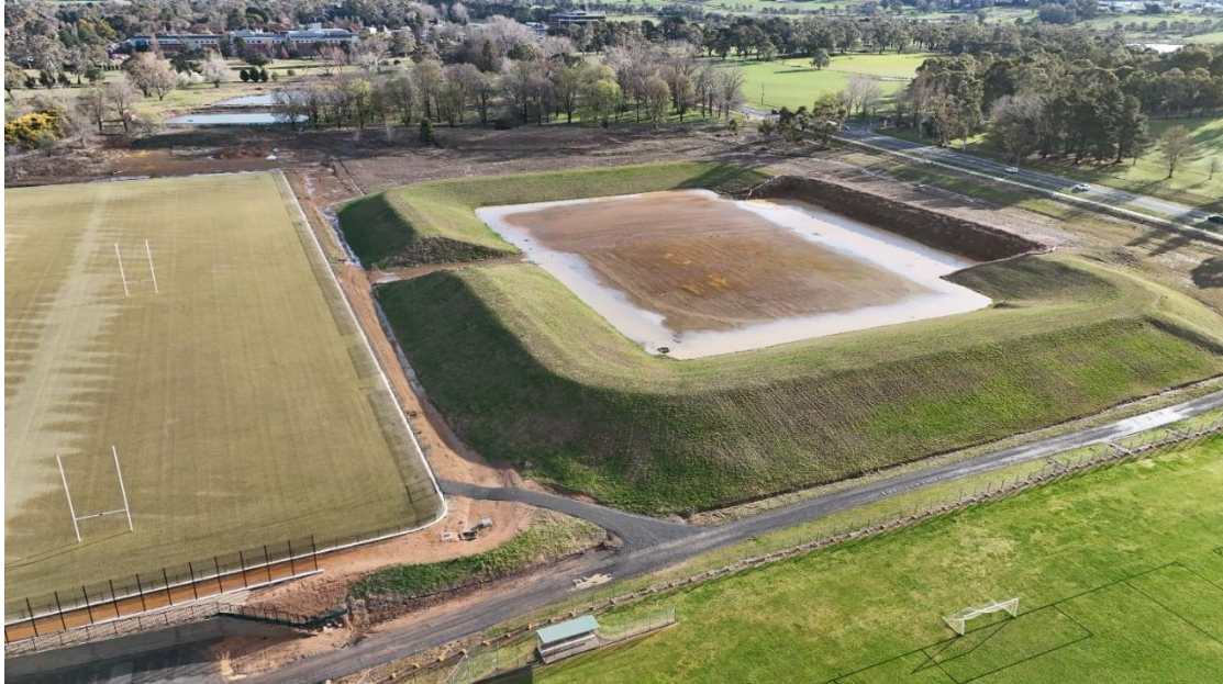
Photo – Sports Precinct – Huntley Road works has commenced onsite.
