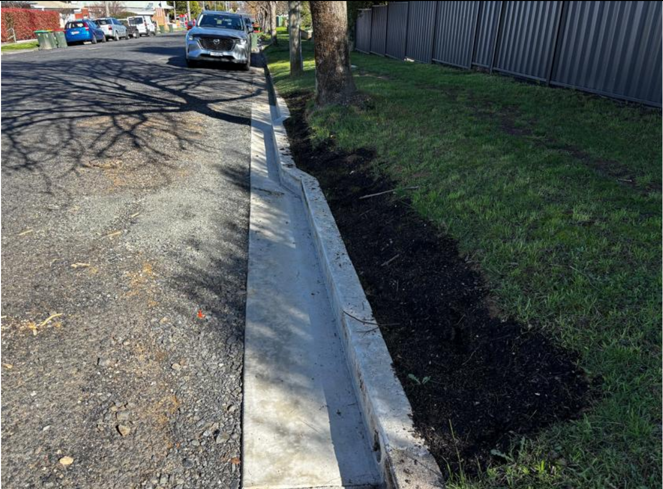
Photo – Kerb reconstruction around street trees in Margaret Street
