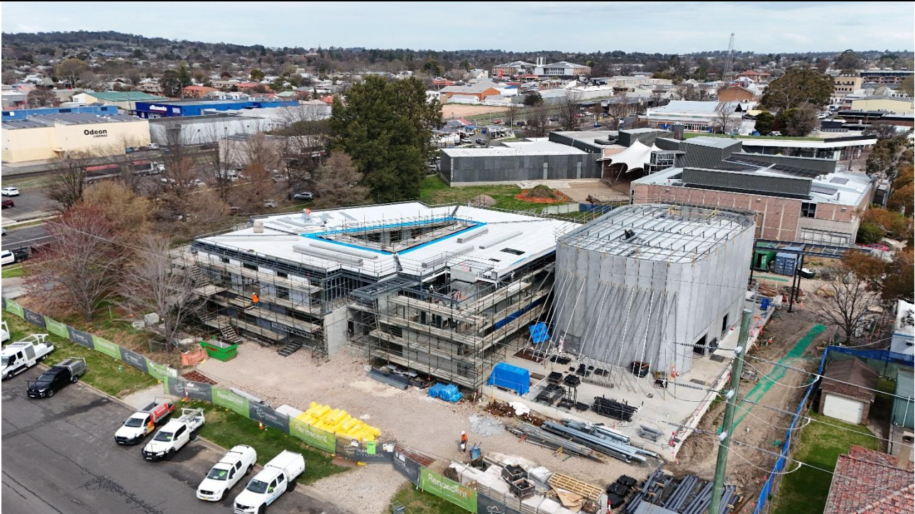
Photo – Construction of Orange Conservatorium and Planetarium – Level 2 structural steel and roofing installation.
