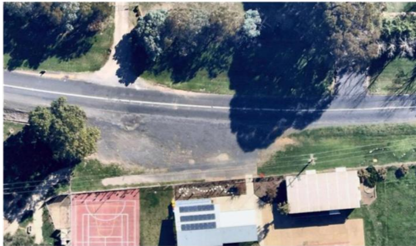
Photo: Pre works being carried out
