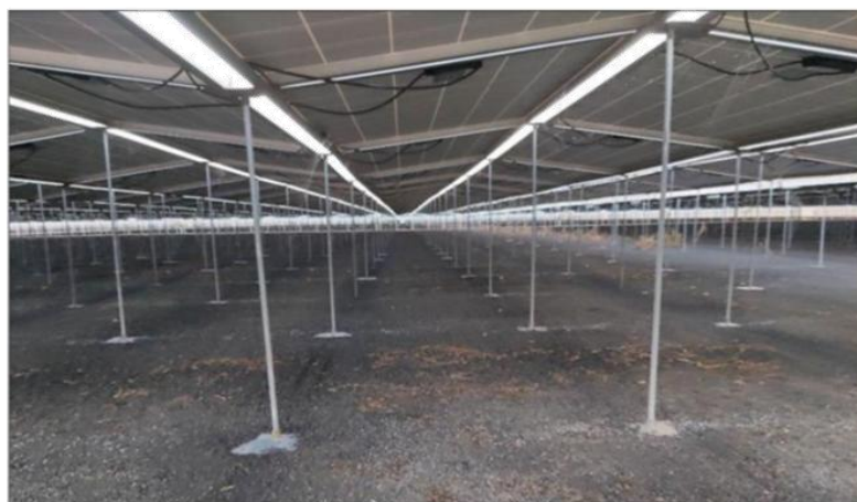
Figure 17 - example of gravel installation beneath PEG system solar panels
