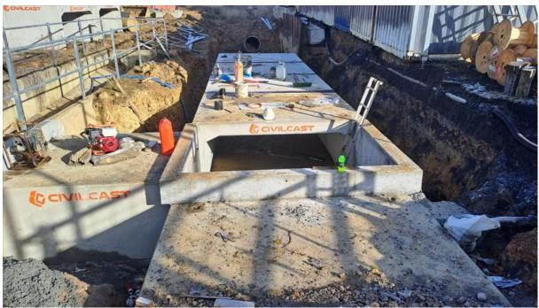
Photo: Concrete box culvert construction
