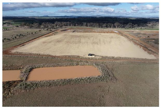
Photo: Topsoil Layer placed on Cells 1 & 2. Construction now complete.
