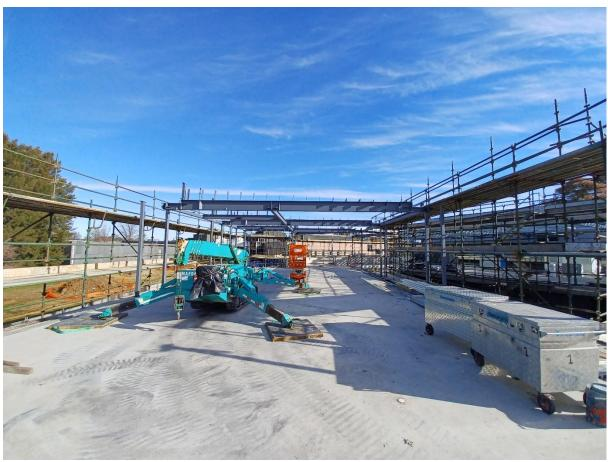
Photo – Construction of Orange Conservatorium and Planetarium – Level 2 structural steel installation
