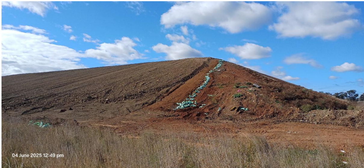
Photo: Revegetation Layer being placed on Cells 1 & 2. Construction now complete.
