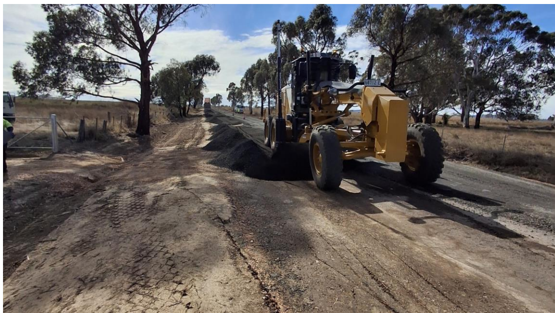
Photo: New gravel being applied to widened road pavement on Aerodrome Road
