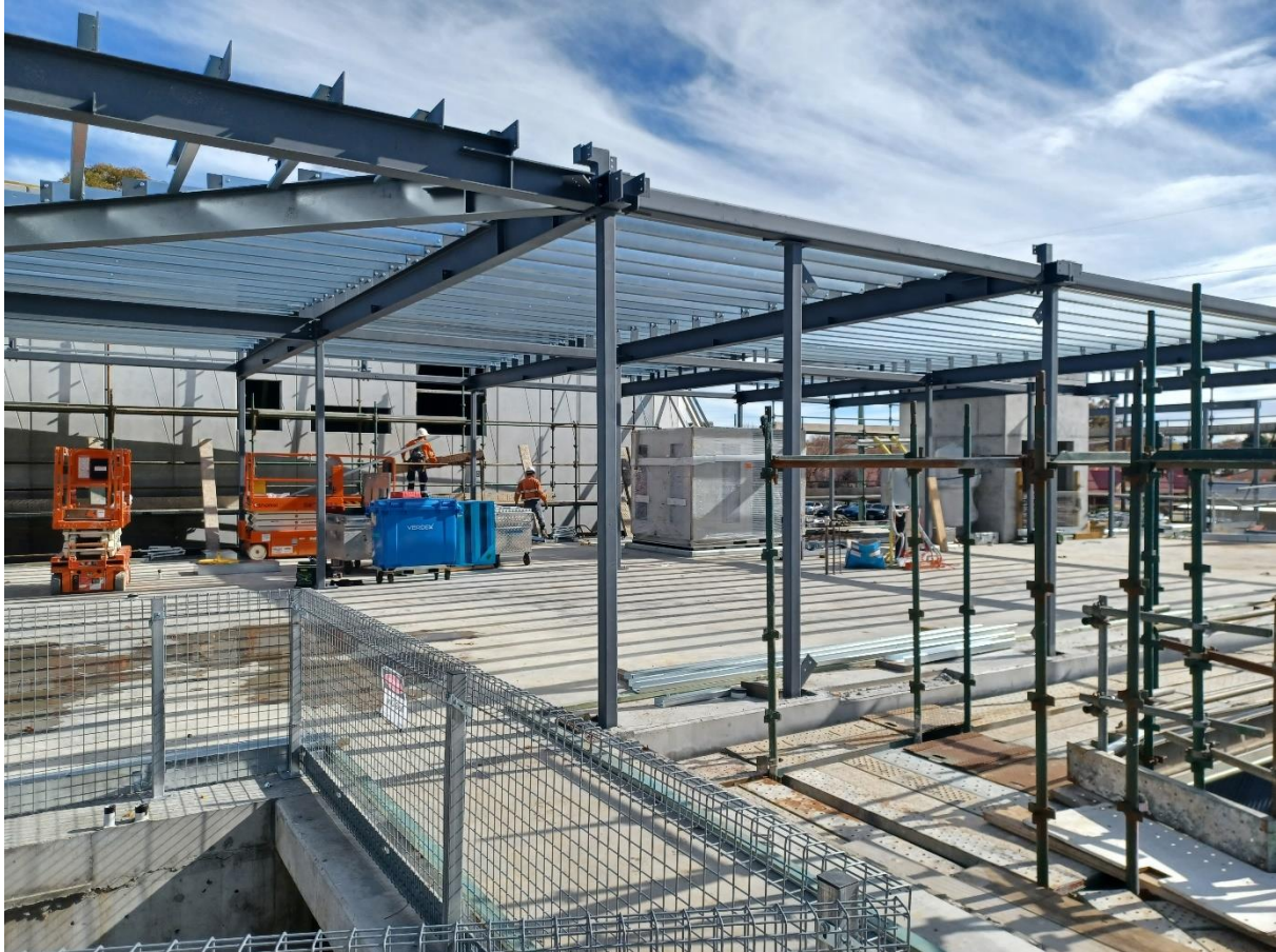
Photo – Construction of Orange Conservatorium and Planetarium view of the structural steel install on level 2.
