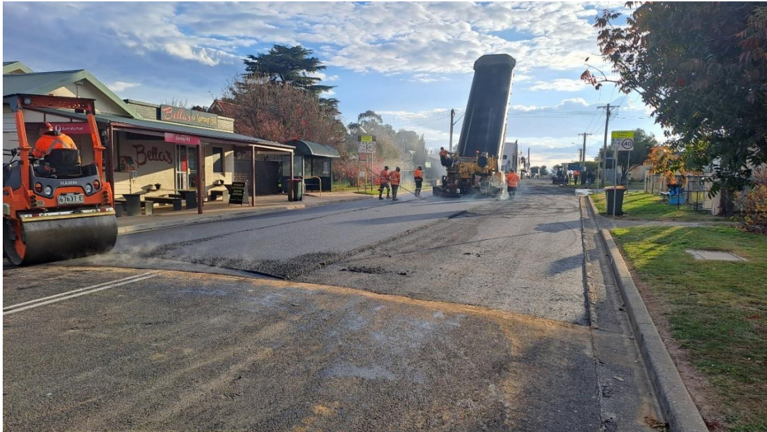
Photo: Asphalt being laid on Seaton Street Spring Hill
