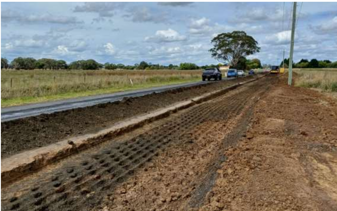
Photo: Excavation of unsuitable base materials in pavement widening area - Forest Road
