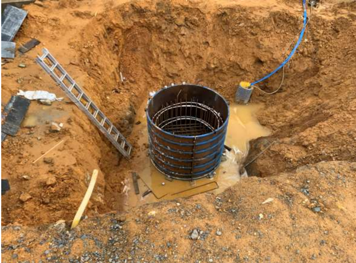
Photo: Grit chamber construction – inlet works
