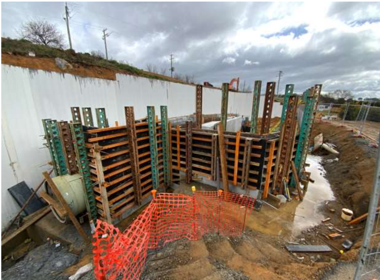
Photo: Formwork for wall construction – inlet works
