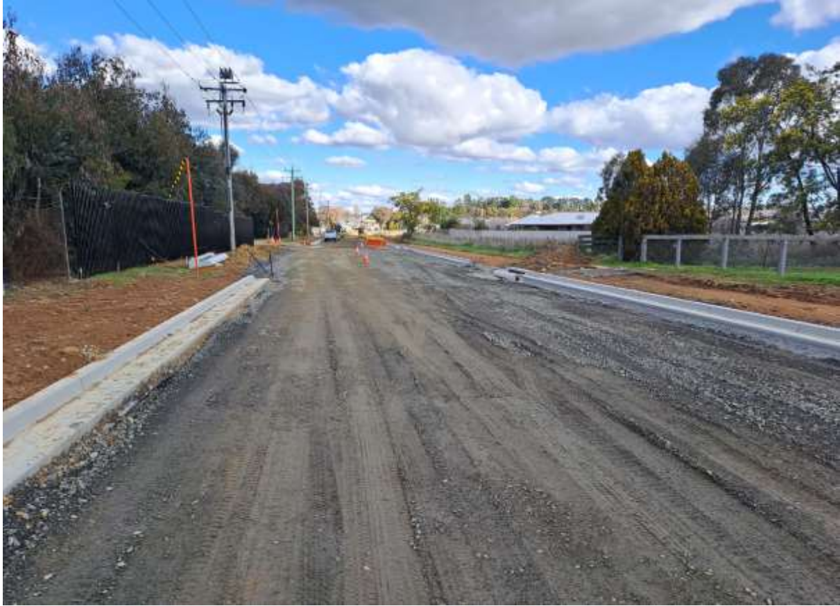
Photo: New kerb and gutter on Clergate Road
