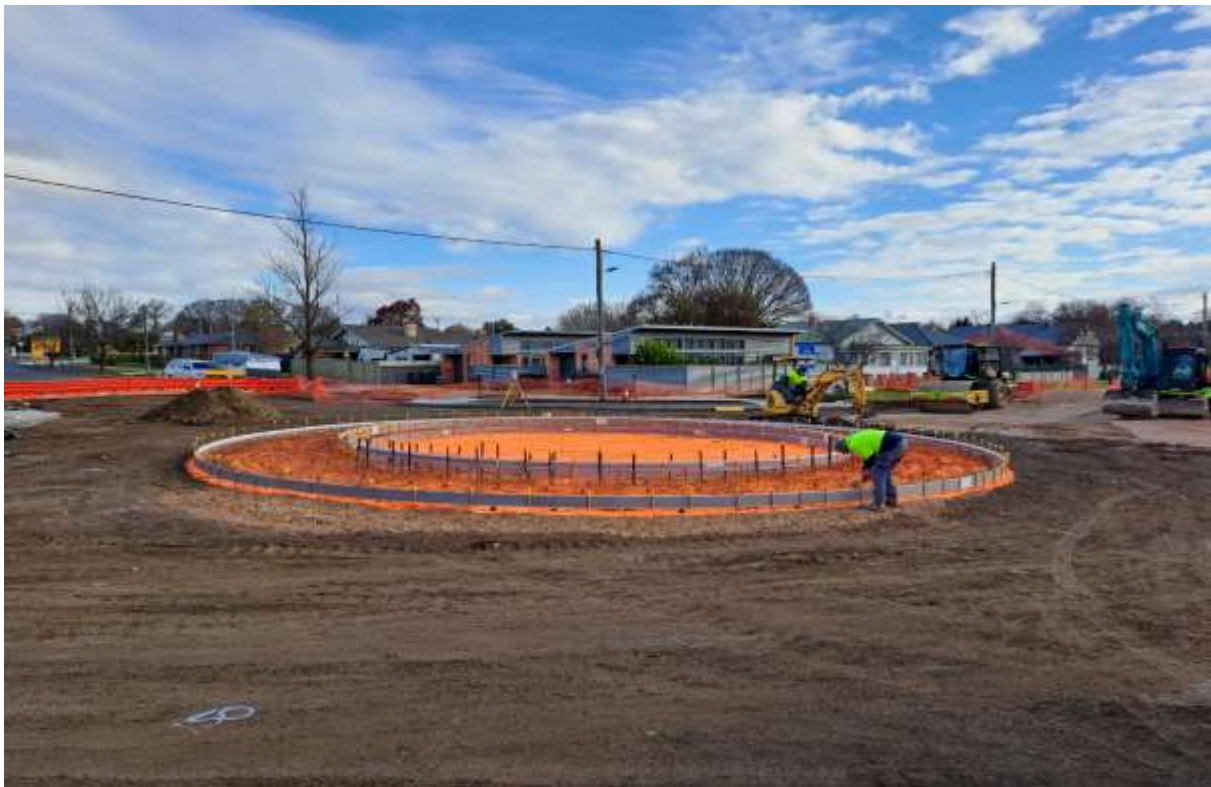
Photo – Formwork and reinforcement for the concrete ring of the roundabout
