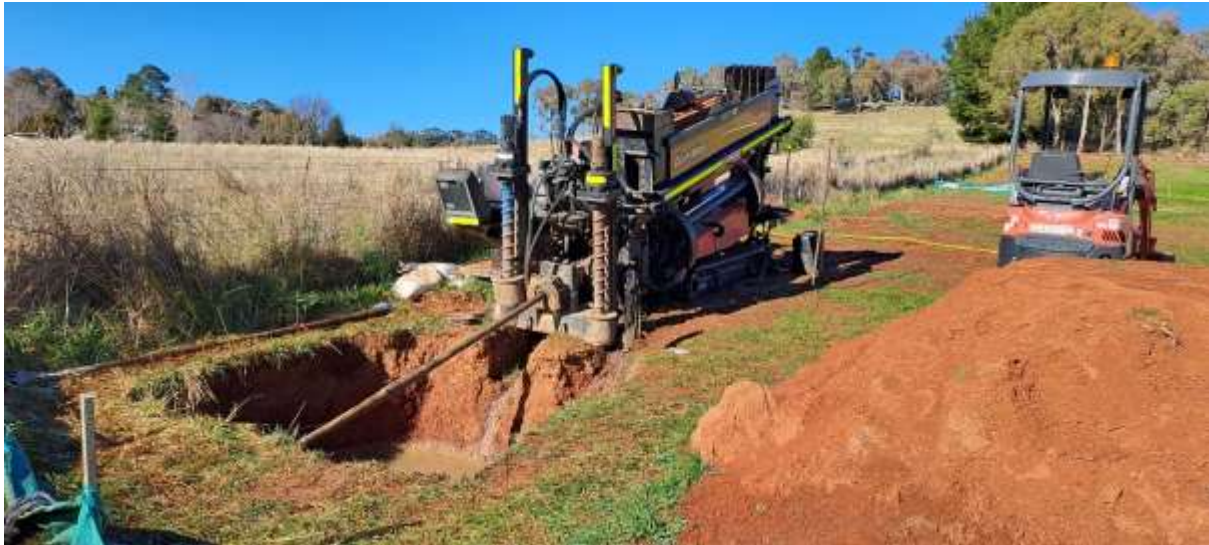
Photo – Under-bore through rock near deer park
