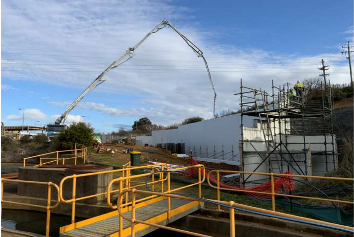
Photo – STP Inlet Works – retaining wall concrete pour 6 June.
