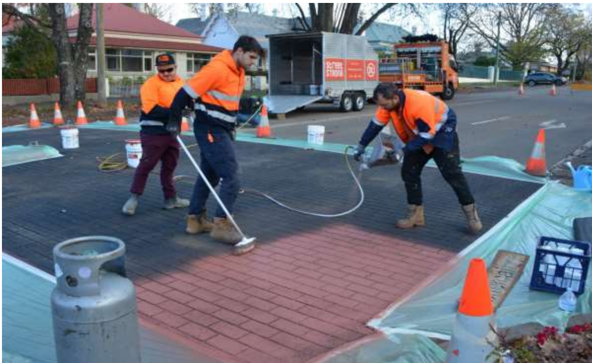
Photo – Contractors painting the stamped asphalt surface
