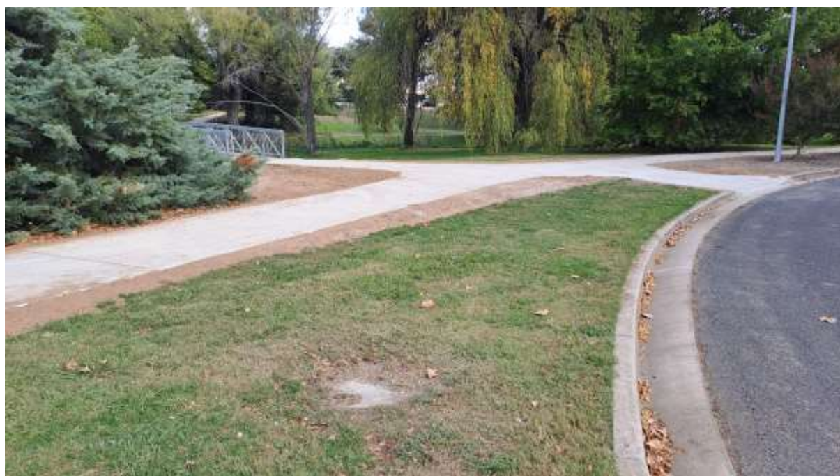
Photo: recently completed section of Moulder Park footpath
