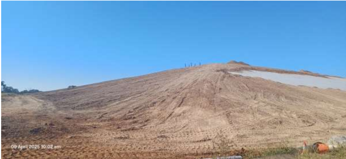
Photo: Revegetation Layer Being place on Cell 1 & 2 Construction
