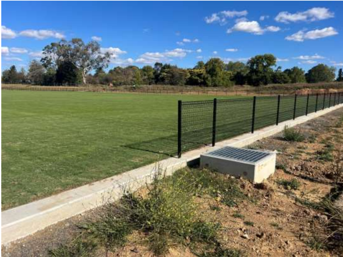
Photo – Turf maintenance ongoing and fencing install around all fields.
