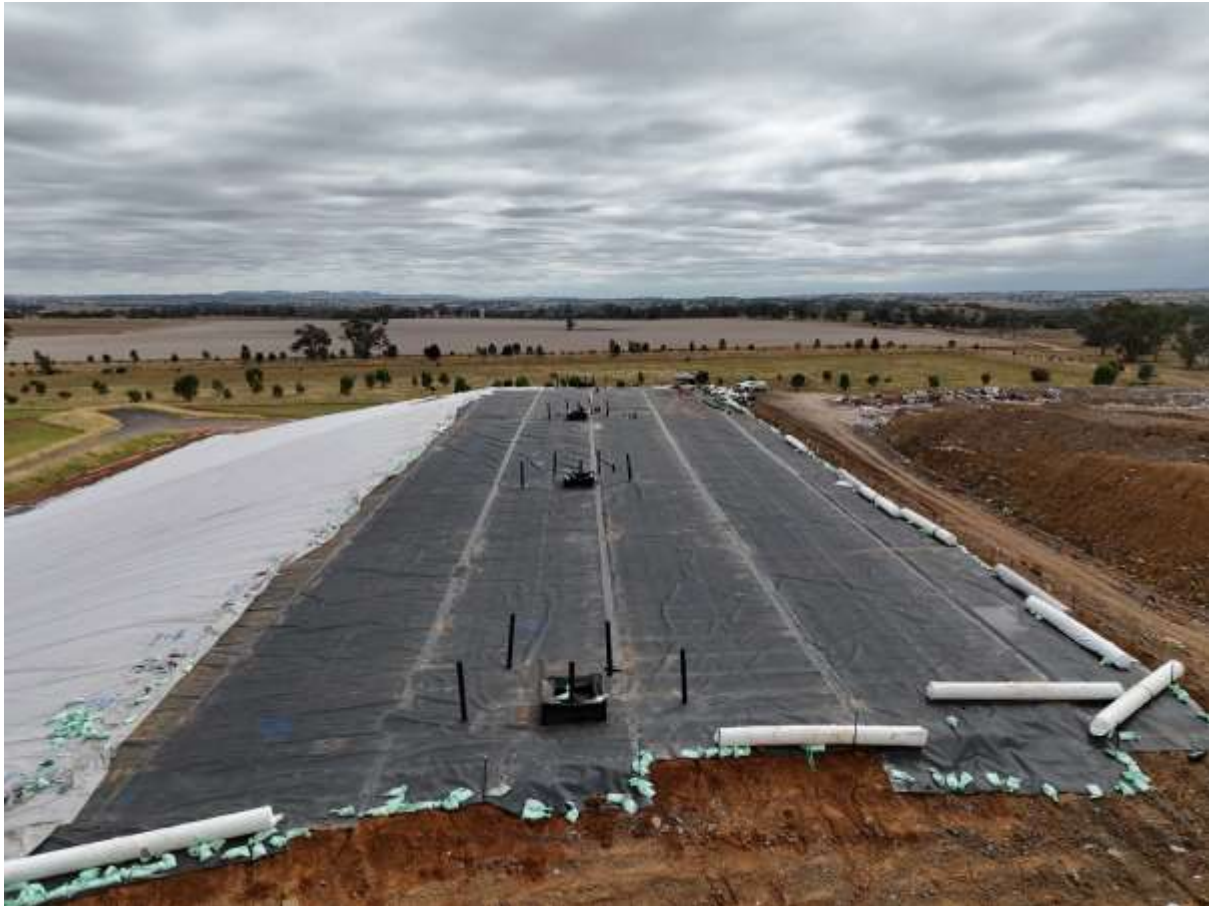
Photo: Completed Clay Seal Bearing Layer Cell 1 & 2 Construction
