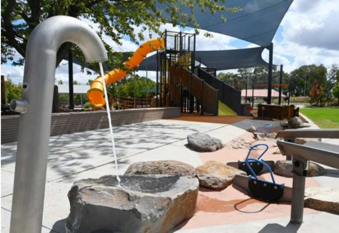
Photo: Adventure Playground – Concrete splash park and equipment being installed
