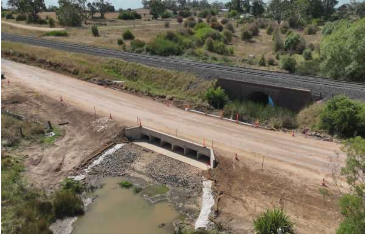
Photo – Road construction over Huntley Road culvert widening
