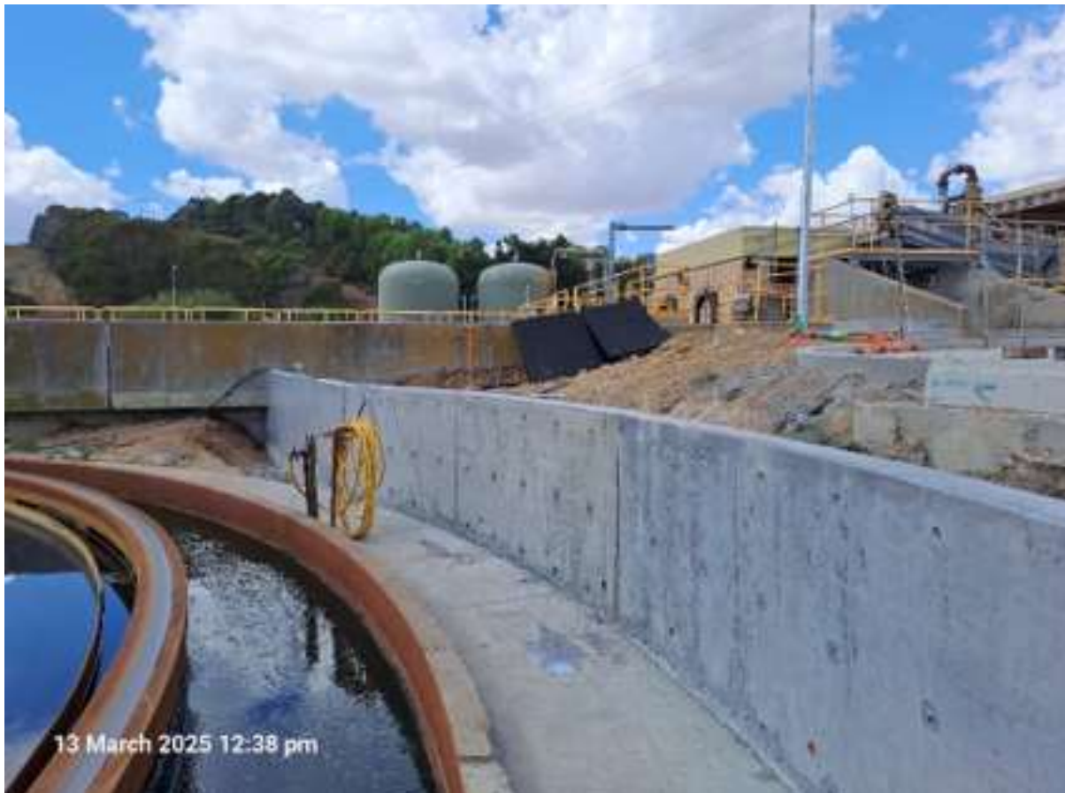
Photo: New retaining wall structure undertaken as a variation to contract
