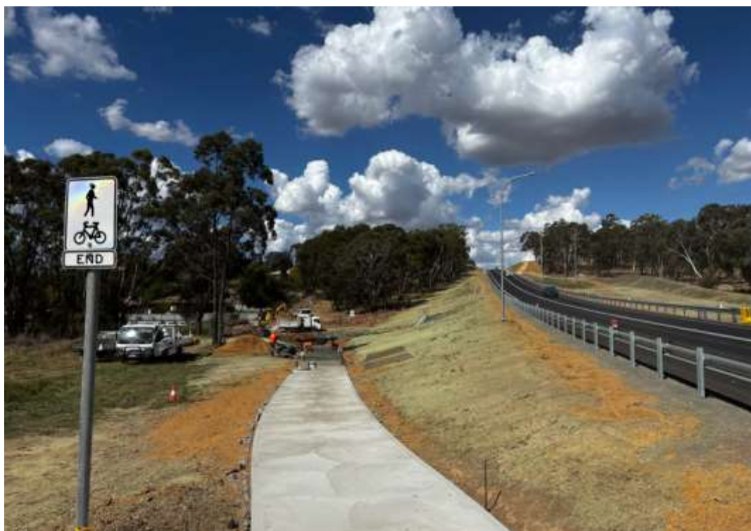
Photo – Shared use path construction between Brabham Way and Sundew Circuit
