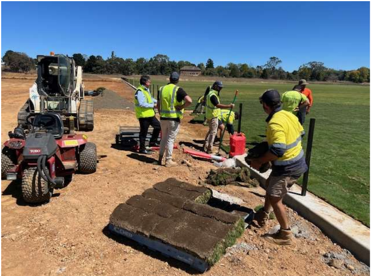
Photo – Last sections of turf being placed on field 5-8
