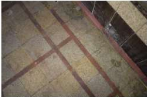
Figure 4.50 | Floor tiling in Public Bar and detail of how it related to the wall tiling. The carpet glue is making it look more yellow than actual colour.
