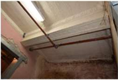
Figure 4.34 | Inside store of Hotel. Pressed metal ceilings and decorative cornicing evident.
