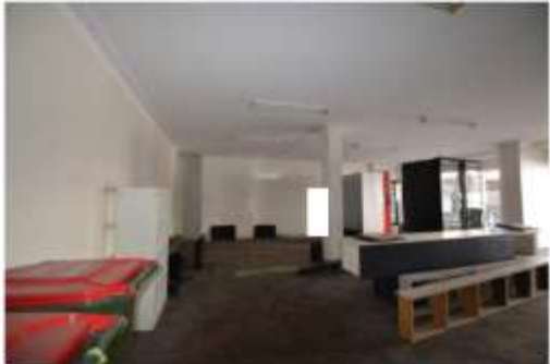
Figure 4.22 | View to the ground floor party wall of No. 249 with Hotel gaming room. An aperture will be put through the 'chimney breast' section, as well as to the right near the front windows to join the two areas.
