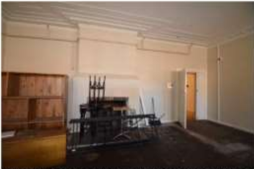
Figure 4.51 | First floor function room. Carpet removed due to water damage from a burst water pipe. Early ceiling and fireplace.
