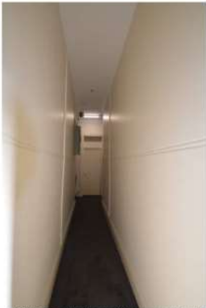
Figure 4.59 | Corridor leading south from women's bathroom above. 3 x doors to new women's bathroom facilities and fire egress to be installed in wall at right.
