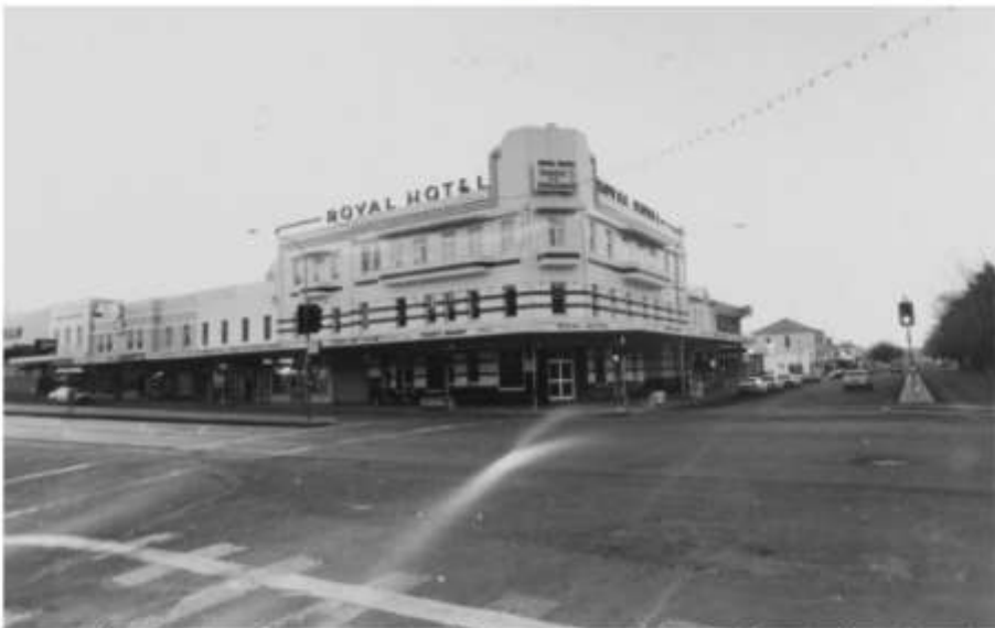
Figure 3.22 | A 1980s view of the Royal Hotel , Tooth & Co. is no more, and the hotel advertises for Tooheys. The corner splay door has been replaced and tiling changed around it. The streamlines have been painted in a dark colour at first, second floors and the parapet. [CWL: Glen Griffith, Royal Hotel Orange , 1980s, photo 800978 ]
