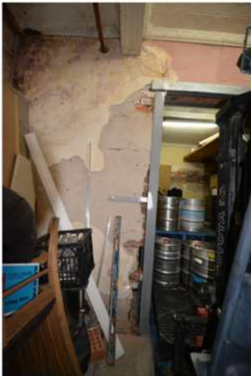
Figure 4.36 | Inside store of Hotel. Exposed sandstock bricks and pressed metal ceilings evident.
