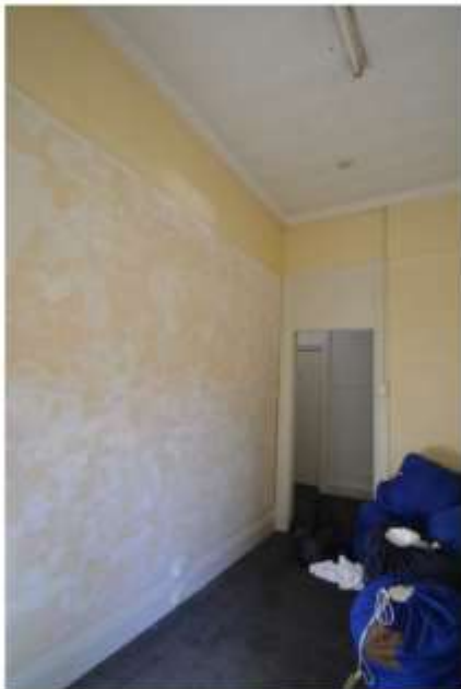
Figure 4.60 | Room/corridor to fire egress stairs at northwest rear corner. Women's bathrooms to be installed in here. The door architraves to remain and be infilled with lightweight material. Ceiling to be protected by the installation of a lower suspended ceiling for the bathrooms.
