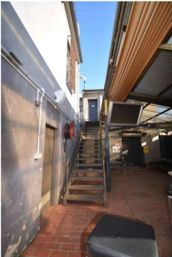
Figure 4.65 | Rear fire stairs to be moved to run east-west, instead of north-south as here.
