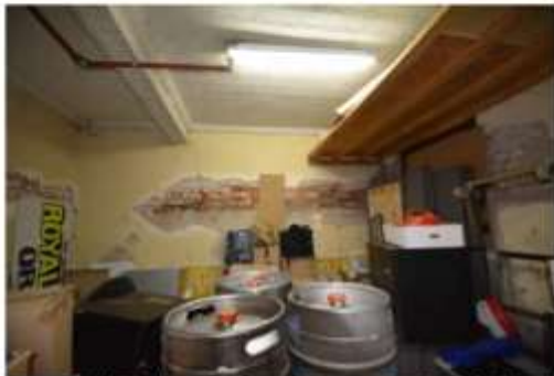
Figure 4.33 | Inside store of Hotel. Exposed sandstock bricks and pressed metal ceilings evident.
