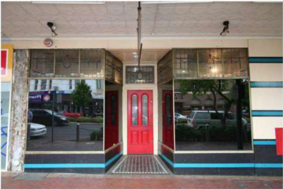
Figure 3.26 | Photo of the part of the Summer Street ground floor façade. Detail of the rendered wall treatment with painted banding at right of image that replaced the vitrolite. [NSW Heritage: Photo by David Scobie, 'Royal Hotel, incorporating Diamond Lil's', State Heritage Inventory database no. 2220480 ]
