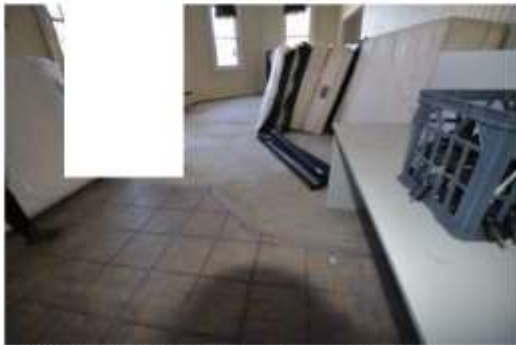
Figure 4.53 | First floor Function room, former saloon bar. Carpet removed due to water damage from a burst water pipe to reveal early tiling, matching that in the Public Bar.
