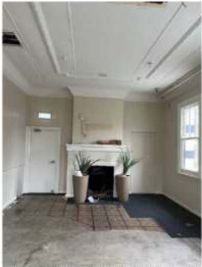
Figure 25 | First floor Function Room significant floor tiling to be left in situ, as is door at right. Bulkhead to be kept at left where part of the wall is proposed for removal.
