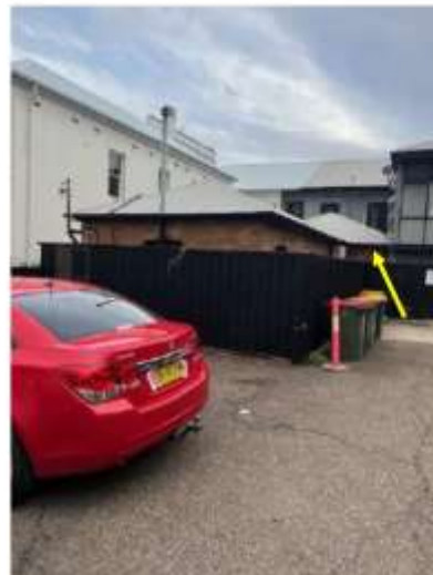
Figure 18 | Sandstock brick rear wing of No. 247. New flat roof and dark batten clad exterior for remnant of rear wing.
