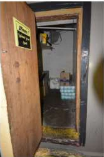
Figure 4.39 | Insulated door to former coolroom, with concrete floor and timber threshold.
