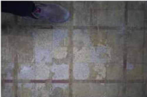
Figure 4.49 | Floor tiling in Public Bar. Original colour and surface evident where the carpet glue has been scraped back. Unfortunatley tiles not extant where the original bar was.
