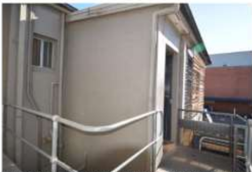
Figure 4.64 | Fire stairs landing will be extended to the wall at right, where a new door will be put in for the Room 18.
