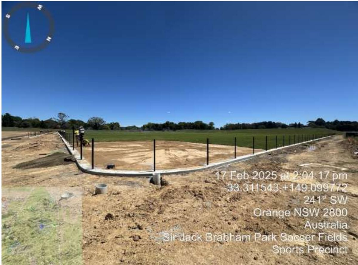
Photo – Installation of fencing and kerbing around the perimeter of the field.
