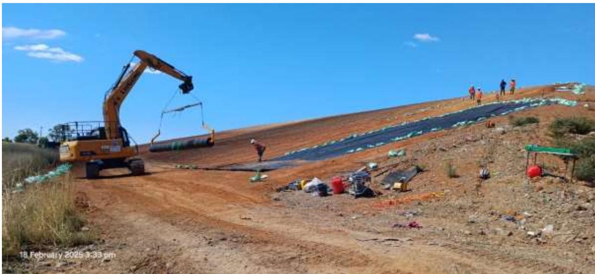
Photo: Completed Clay Seal Bearing Layer Cell 1 & 2 Construction
