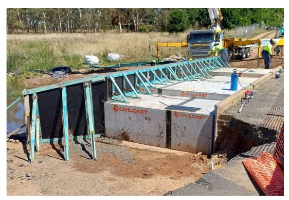
Photo: Concrete works to support road widening
