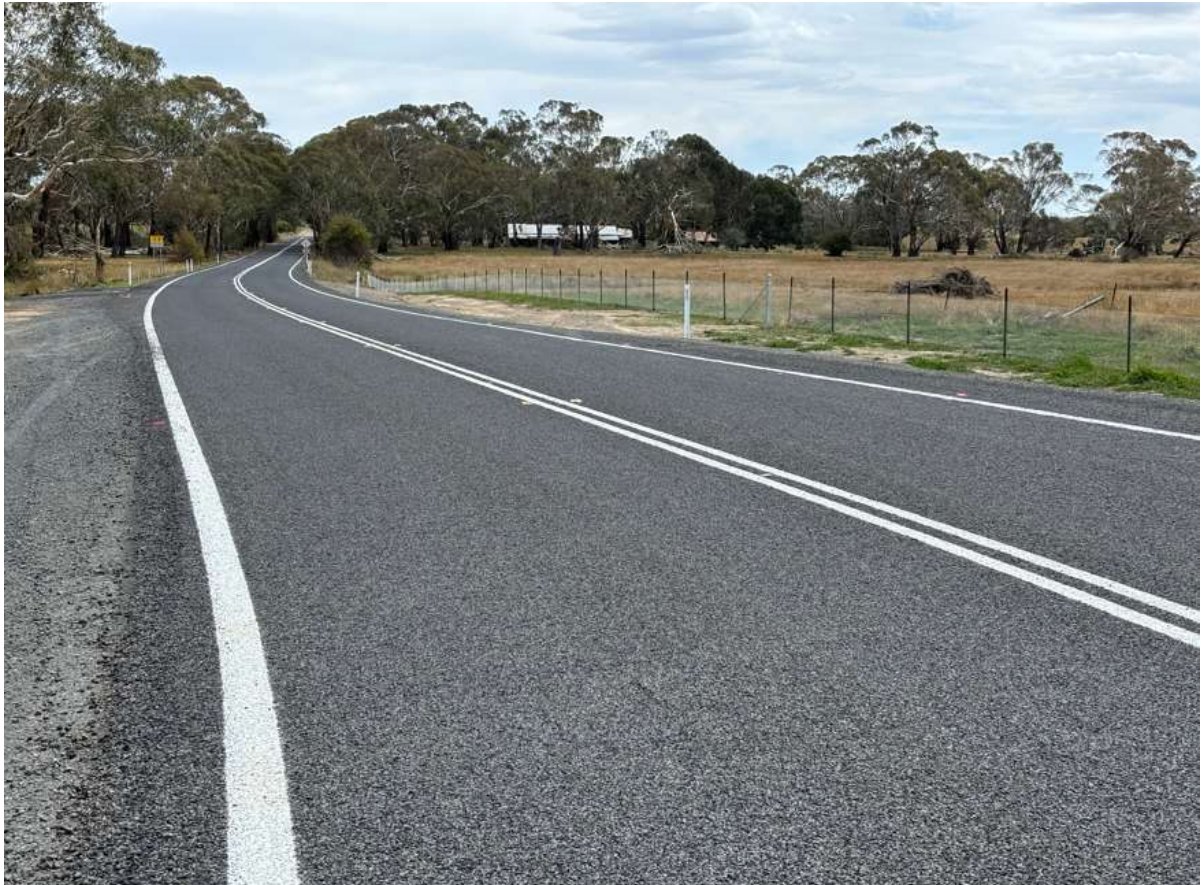
Photo: Pavement upgrade and widening on Huntley Road
