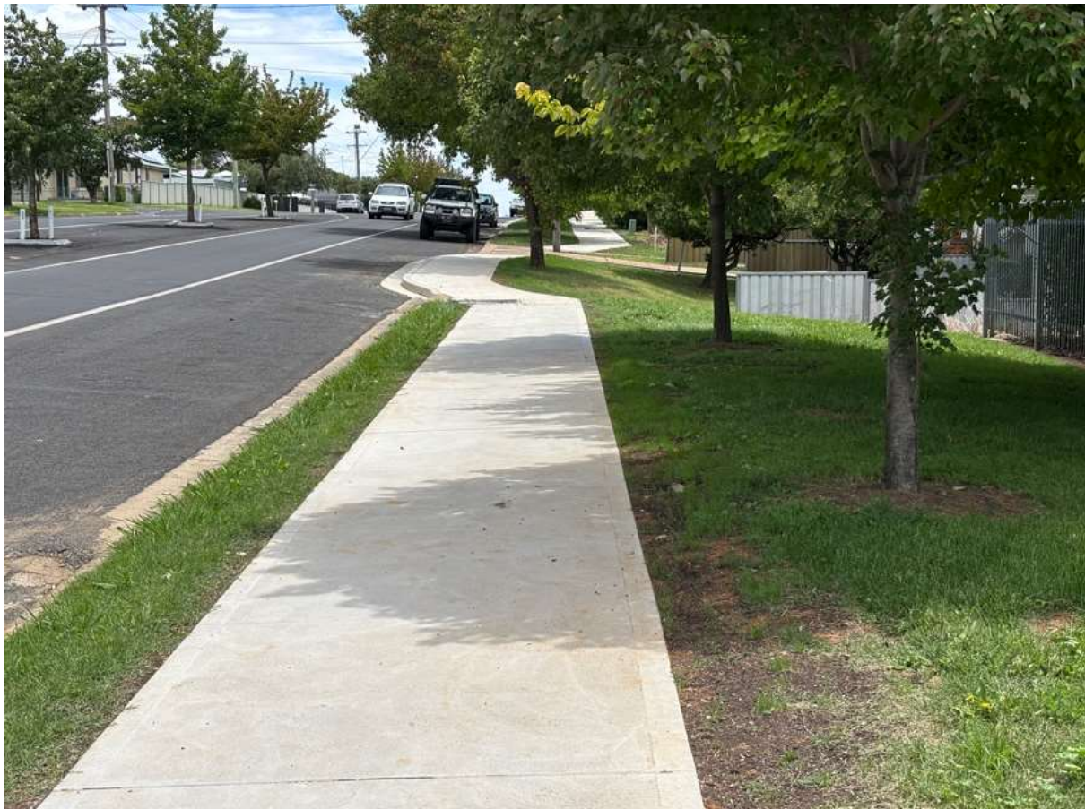
Photo: Completed footpath on Matthews Avenue
