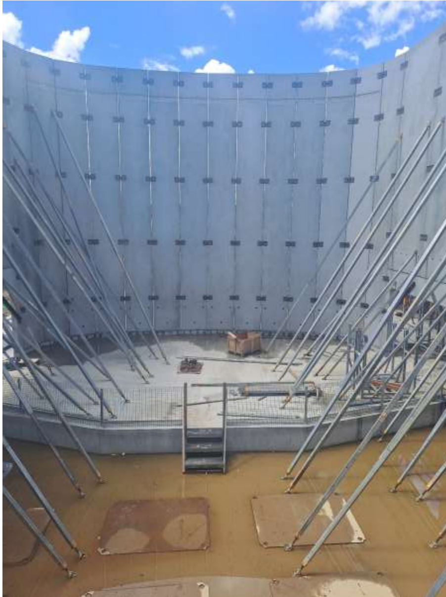
Photo – Construction of Orange Conservatorium and Planetarium internal view of the Recital Hall
