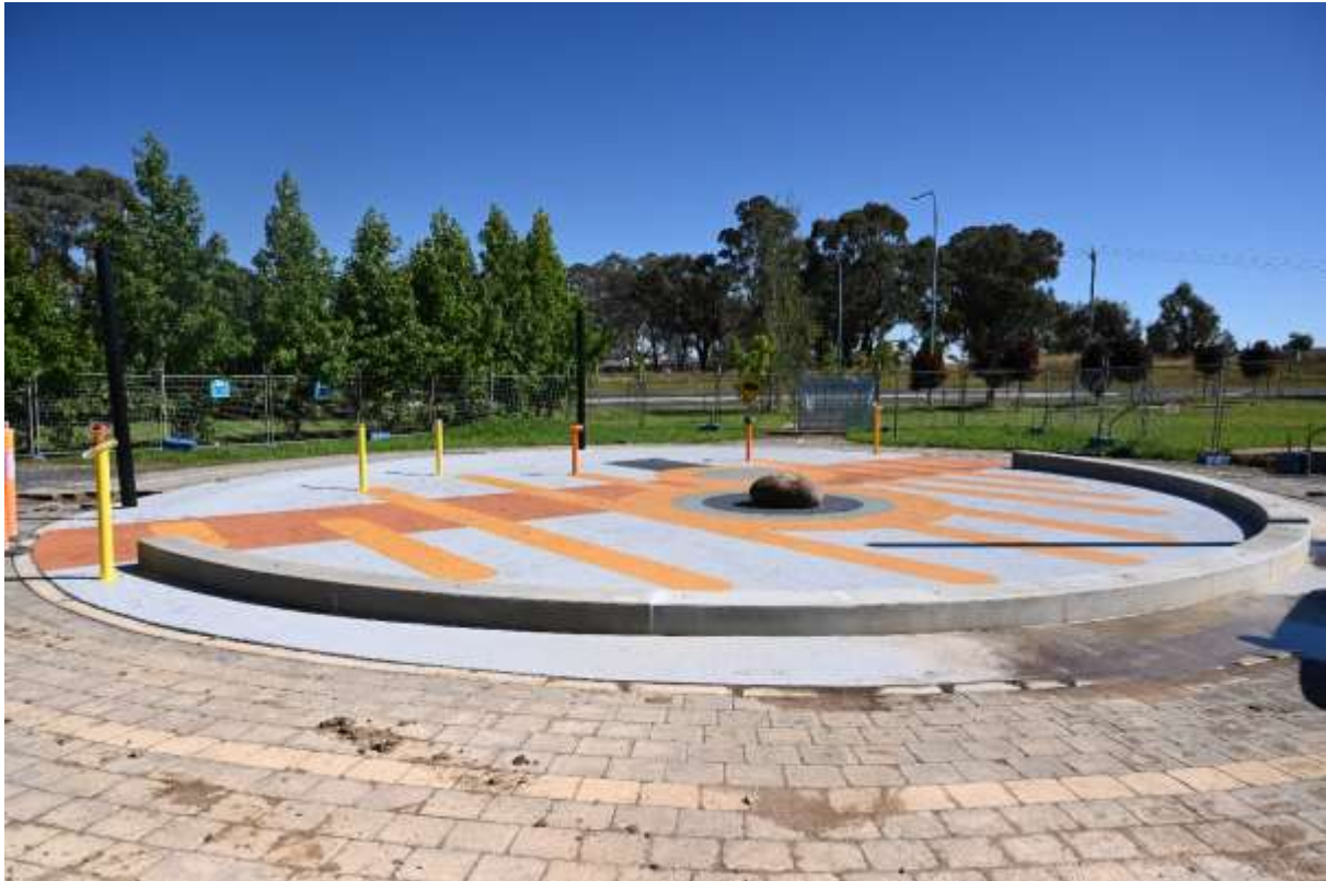
Photo: Adventure Playground – Concrete splash park and equipment being installed
