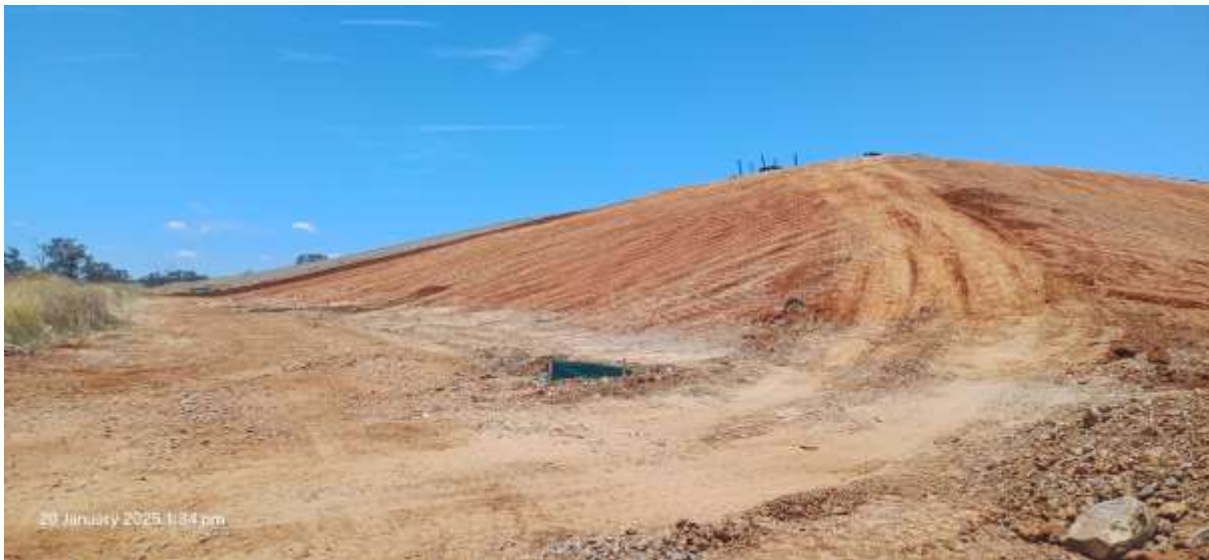
Photo: Completed Clay Seal Bearing Layer Cell 1 & 2 Construction
