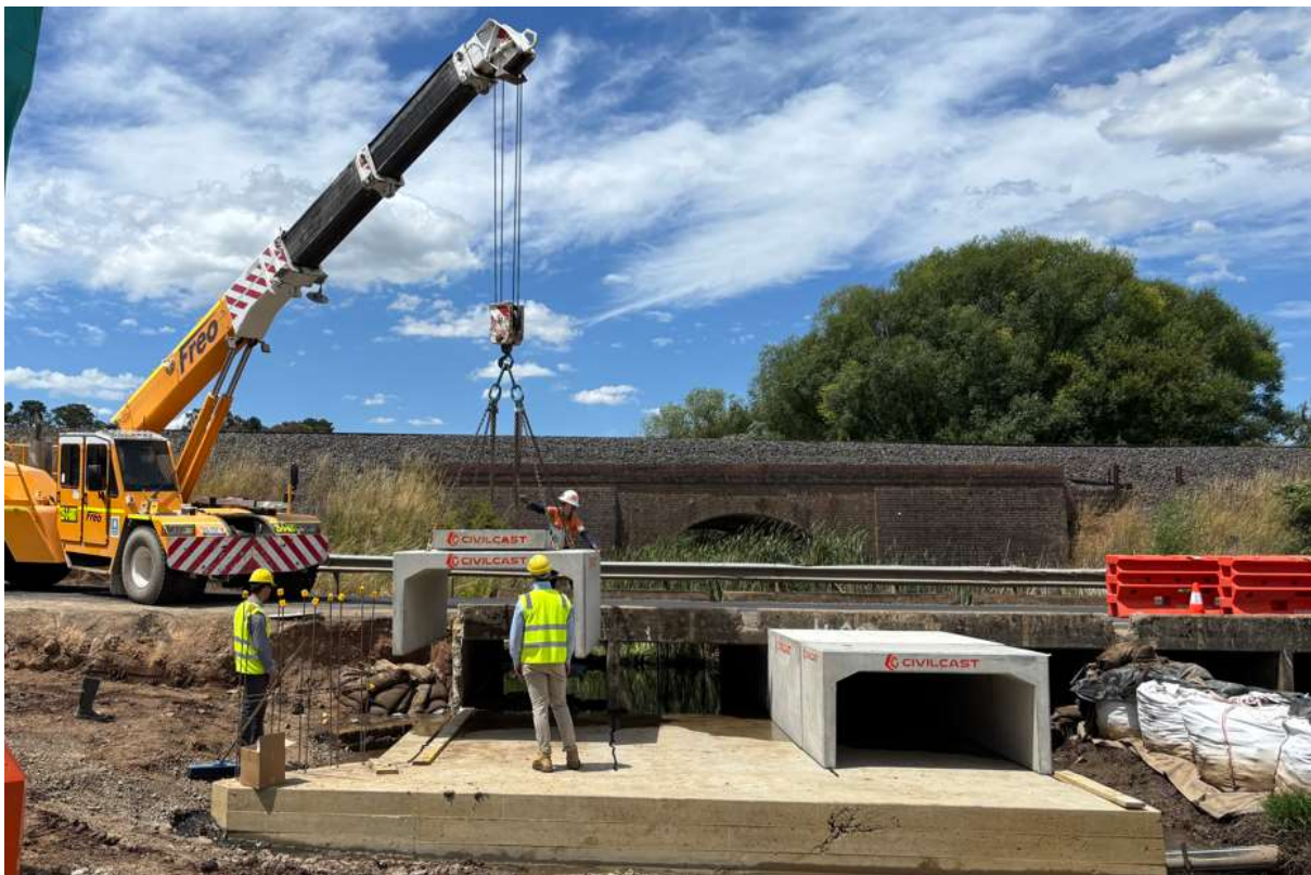
Photo: Box culvert units being placed at Huntley Road
