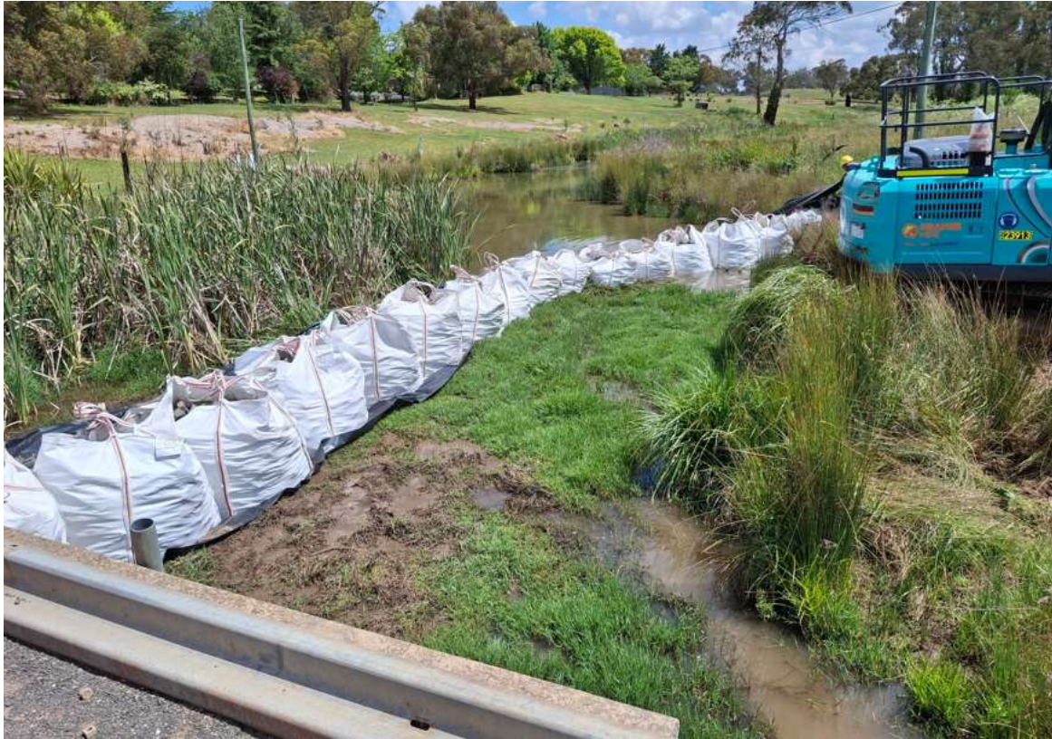
Photo: Clean water diversion being installed in Gosling Creek
