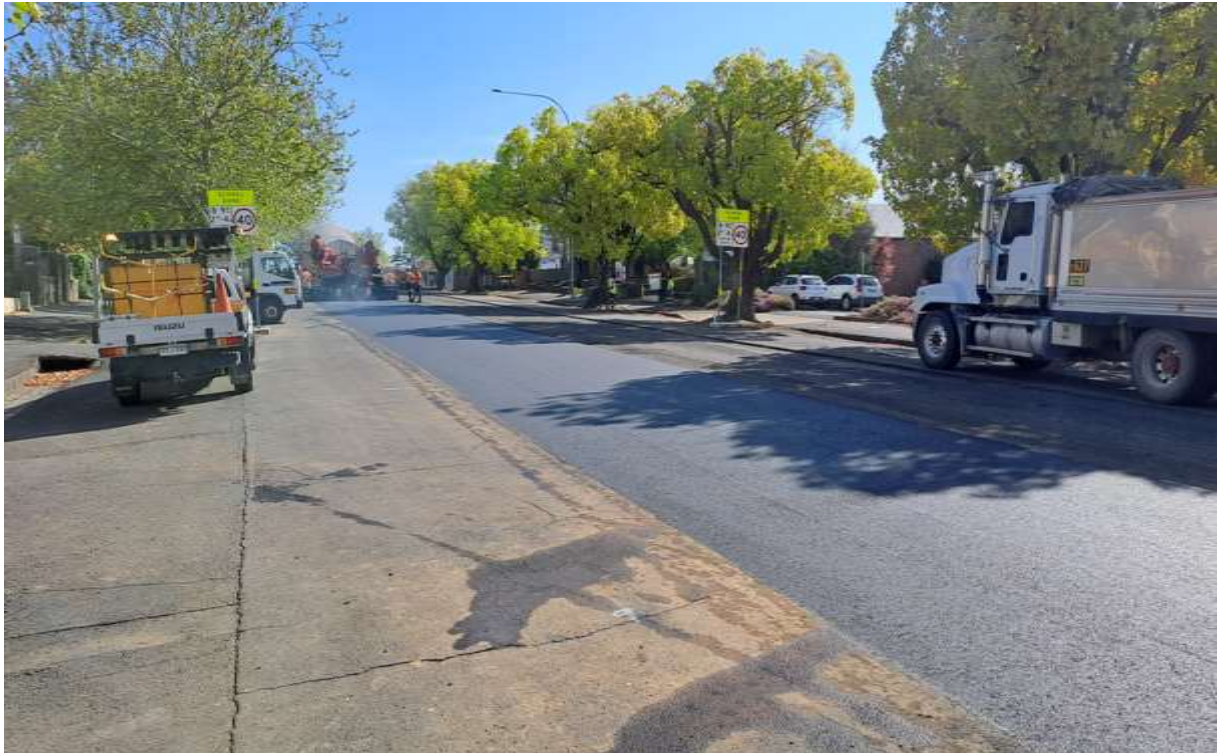
Photo: New asphalt being laid on the travelling lanes in Sale Street following stabilisation of the pavement underneath.
