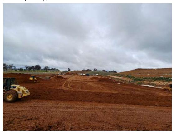
Photo: Installation of clay liners into Cell 4 and batters
