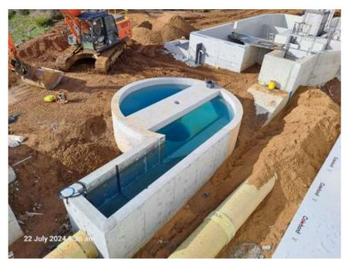
Photo: Contractors undertaking water test on the grit chamber and channel
