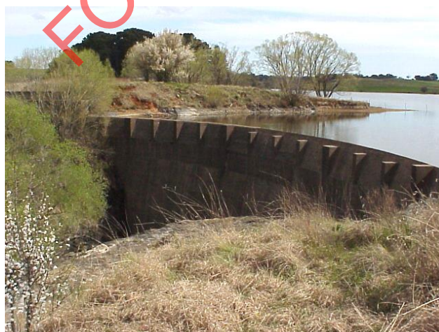
Image 1 - View of concrete arch spillway
