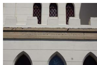
Alterations to the main façade indicating the original / more sympathetic finish and colour of the 1949 Memorial Tower and Porch below later applied signage together with remnant lettering (Source : Christo Aitken + Associates)
