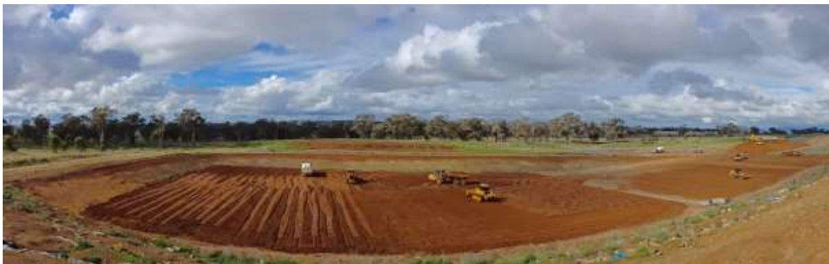
Photo – Construction of new waste cell and clay liner being placed.
