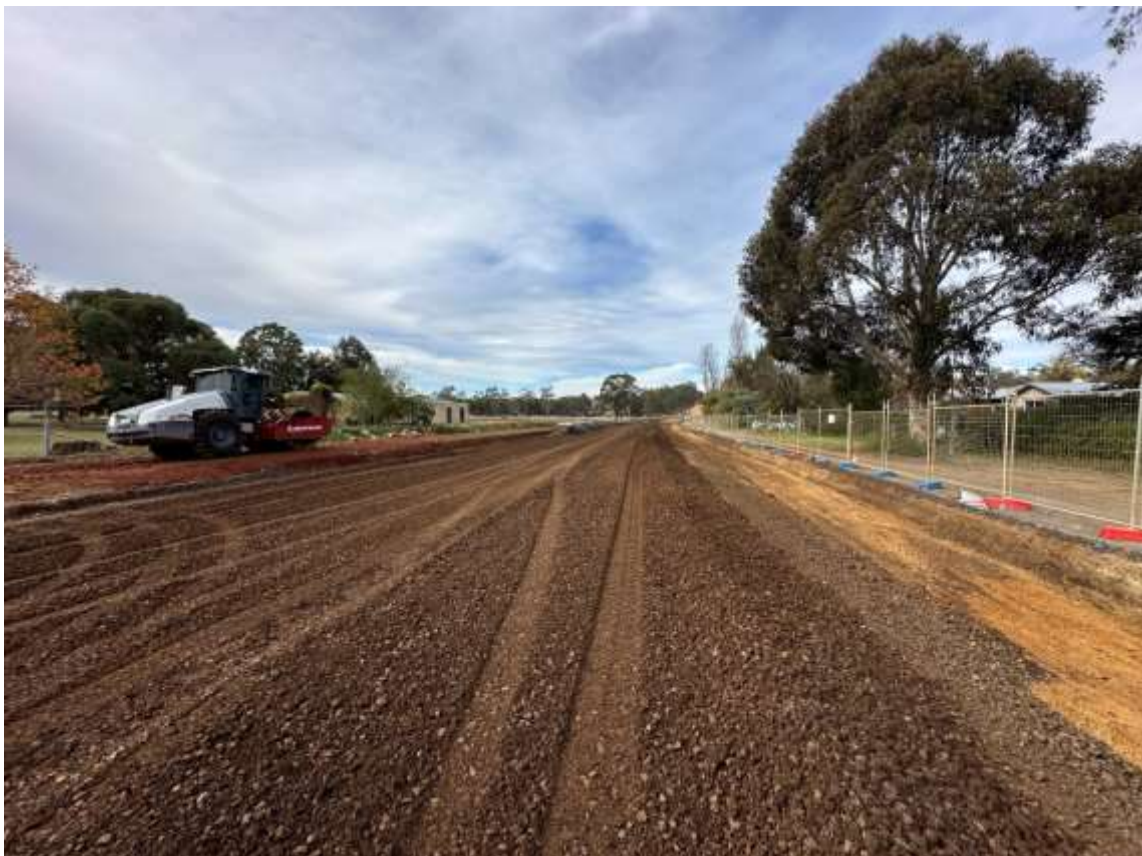
Photo – Southern Feeder Road
