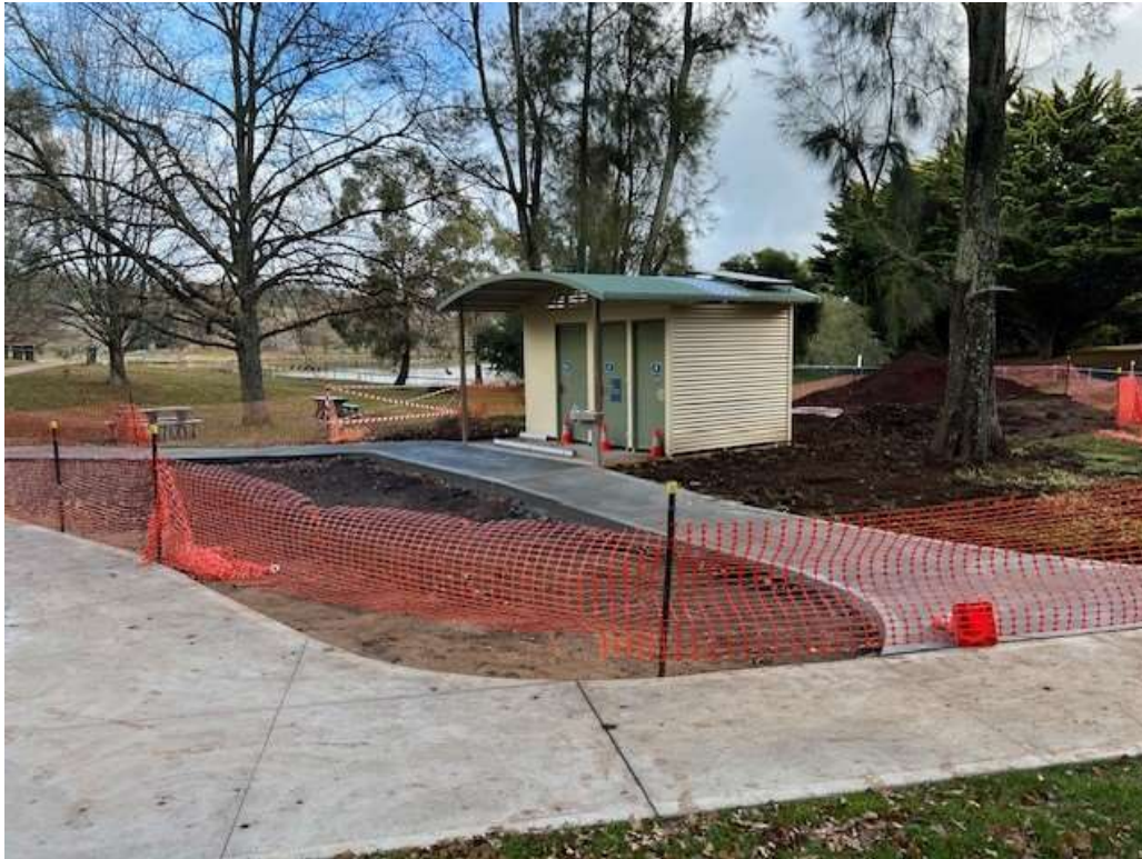
Photo – Lake Canobolas toilet facilities
