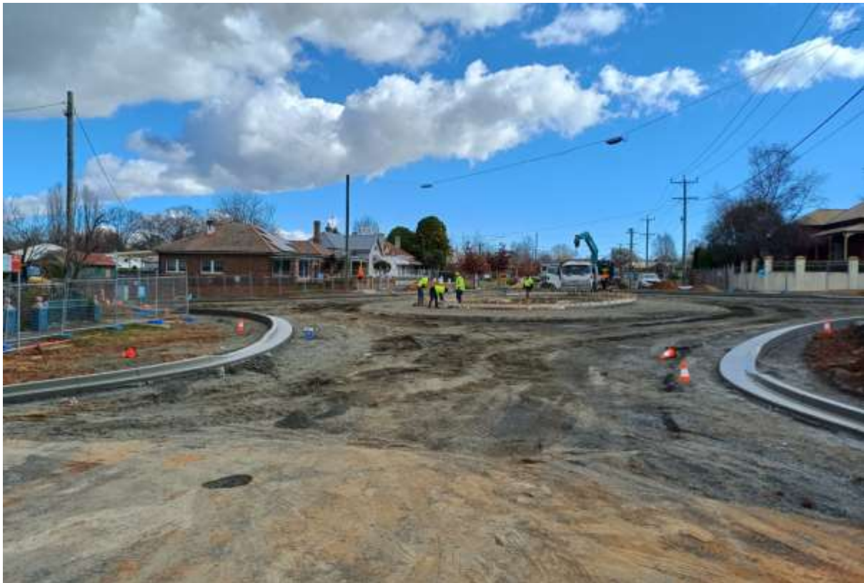
Photo – Roundabout progress with freshly poured kerbs
