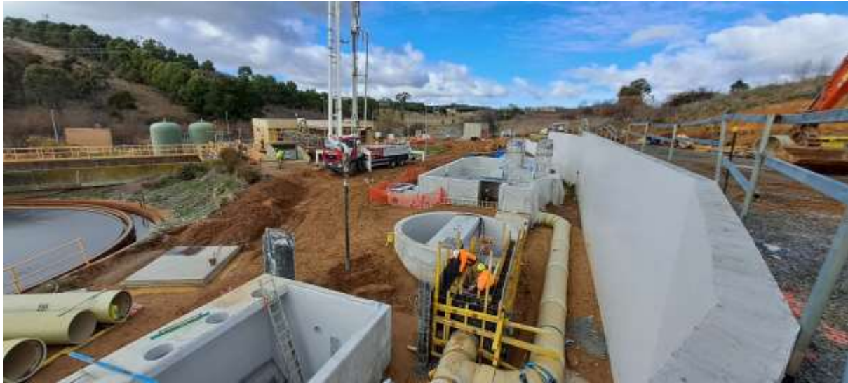
Photo: Contractors about to pour grit chamber channel
