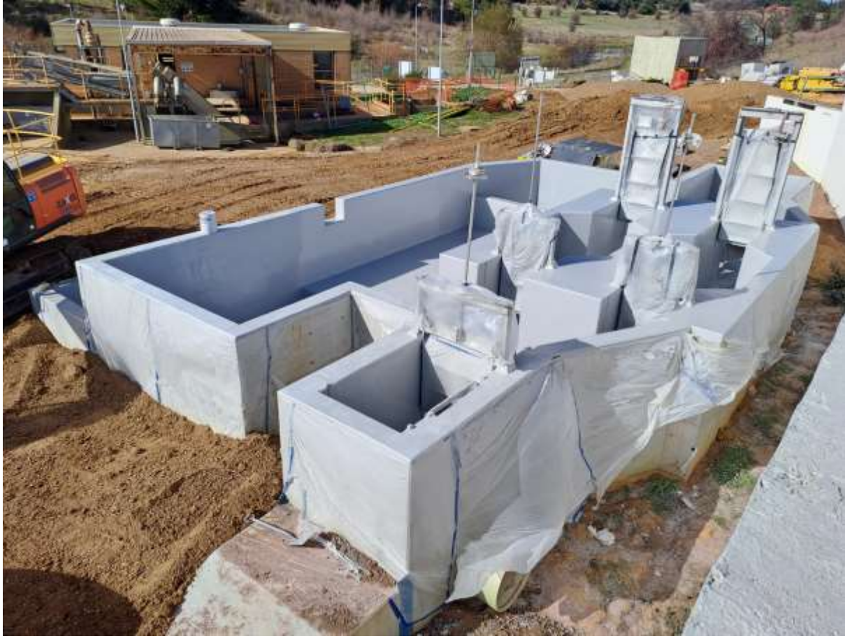
Photo – Inlet structure - epoxy coating
