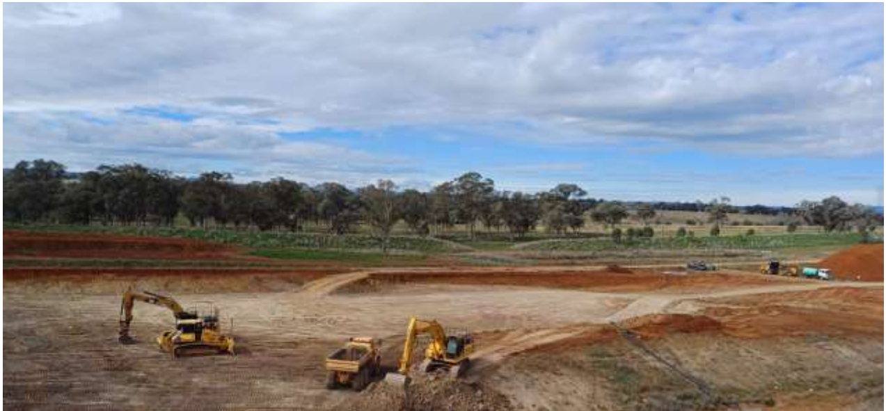
Photo – Construction of new waste cell
