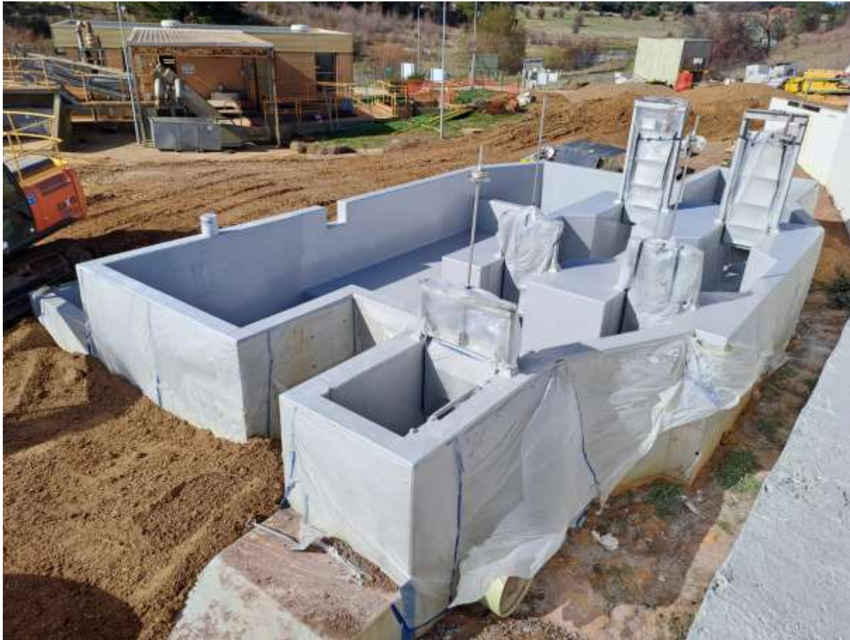
Photo – Inlet structure - epoxy coating
