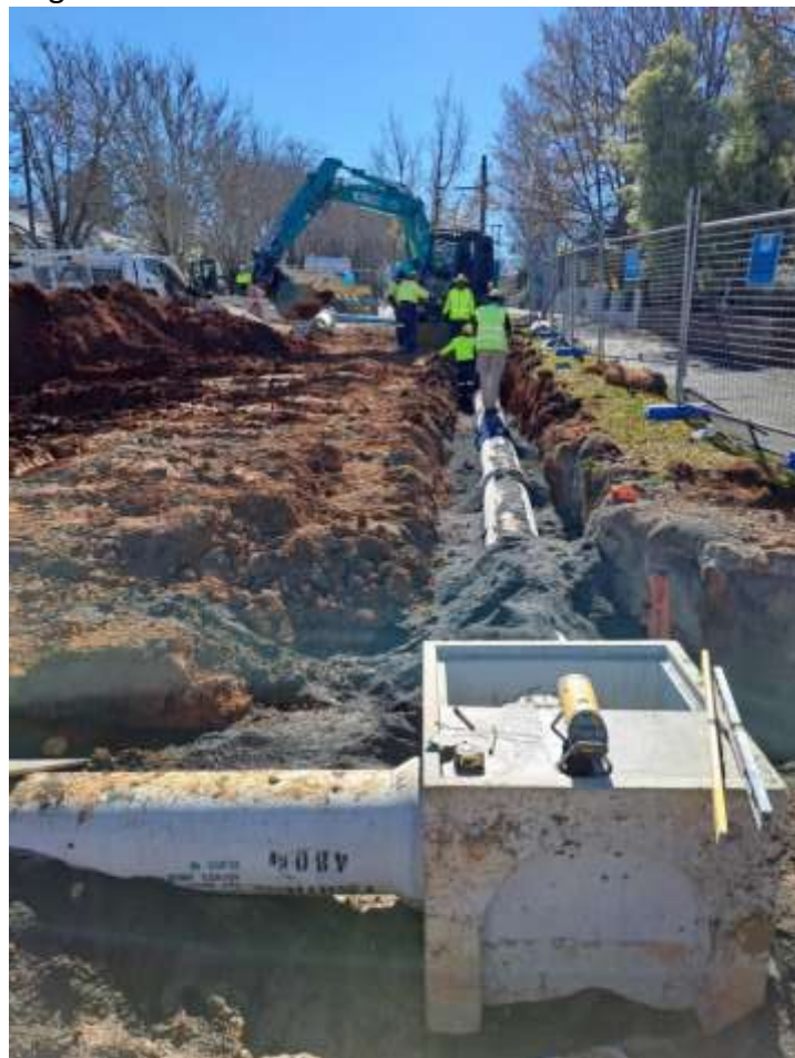
Photo – Stormwater drainage upgrades at Hill and Moulder Street
