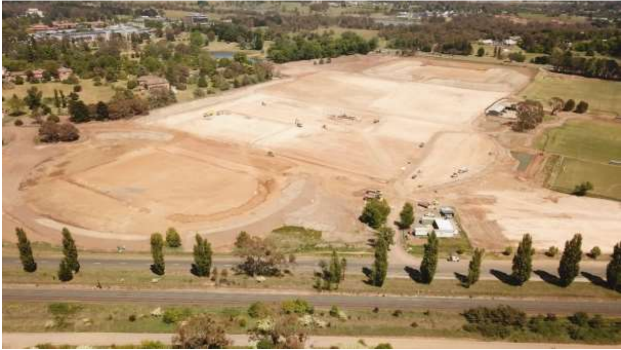
View of completed earth works from Athletics Precinct (Huntley Road) side
