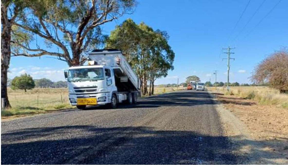
Photo – Sealing completed road works on Forest Road
