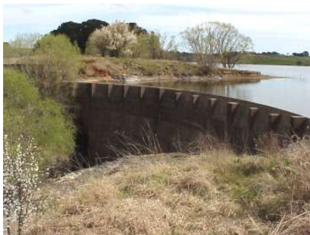
view of concrete arch spillway
