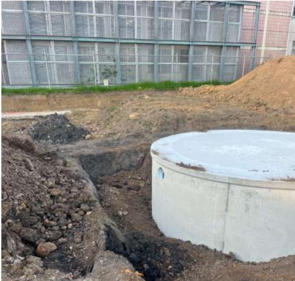
Week Ending 1 st March – Backfilling of Rainwater tank
