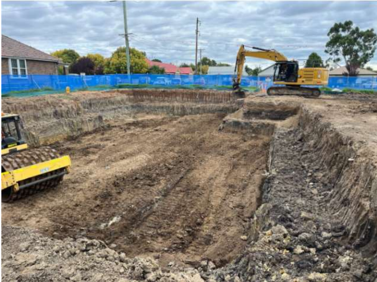
Week Ending 15 th March – Excavation of Borrow Pit
