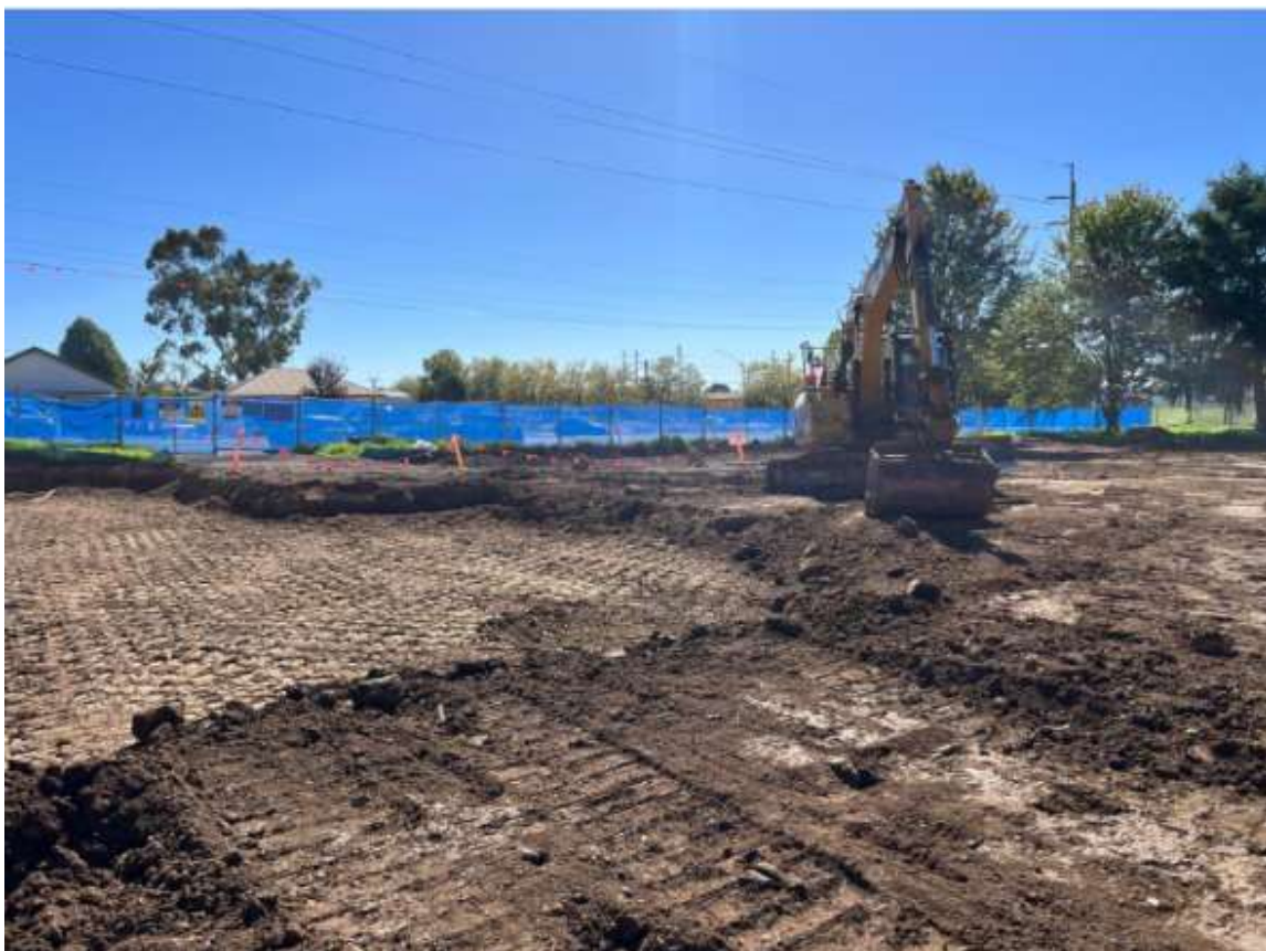
Week Ending 22 nd March – Backfilling borrow pit.
