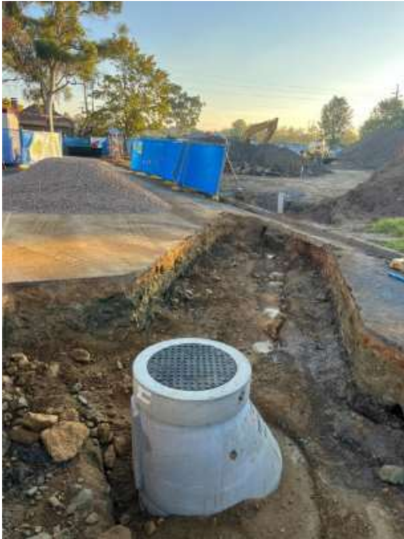
Week Ending 29 th March - new sewer connection to site.
