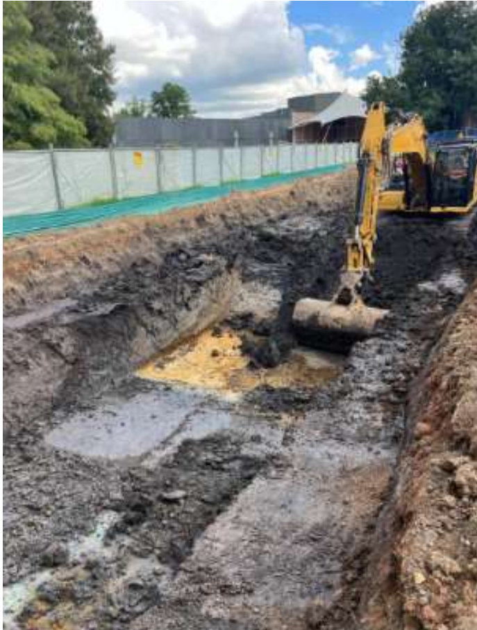
Week Ending 23 rd February – Excavation of soil to be remediated.
