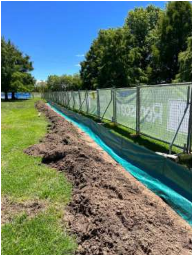
Week Ending 26 th January – Site Facilities and Sediment Fence Installation
