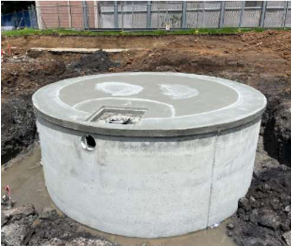
Week Ending 16 th February – Rainwater tank installation
