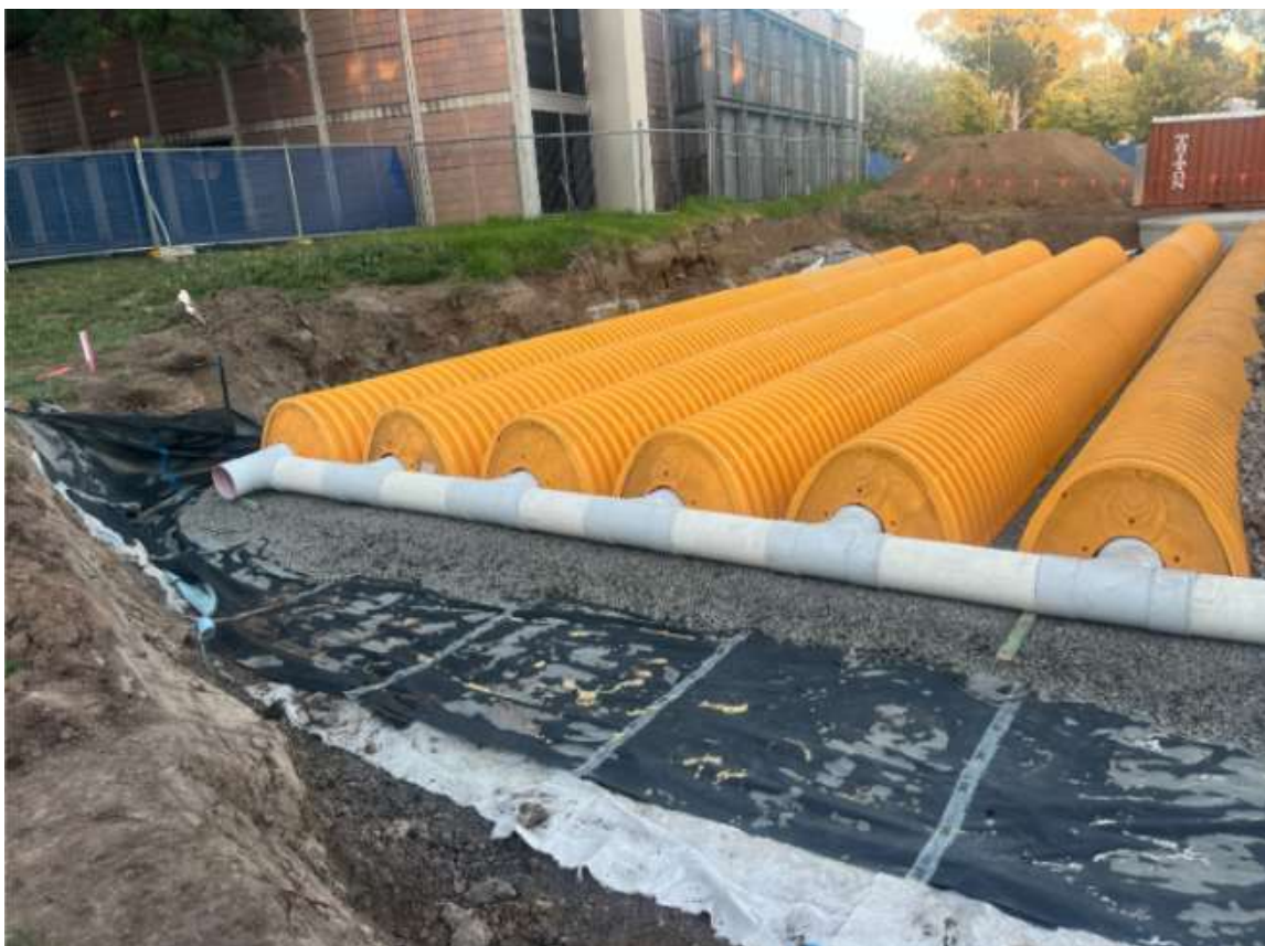
Week Ending 8 th March – Installation of on-site detention tank
