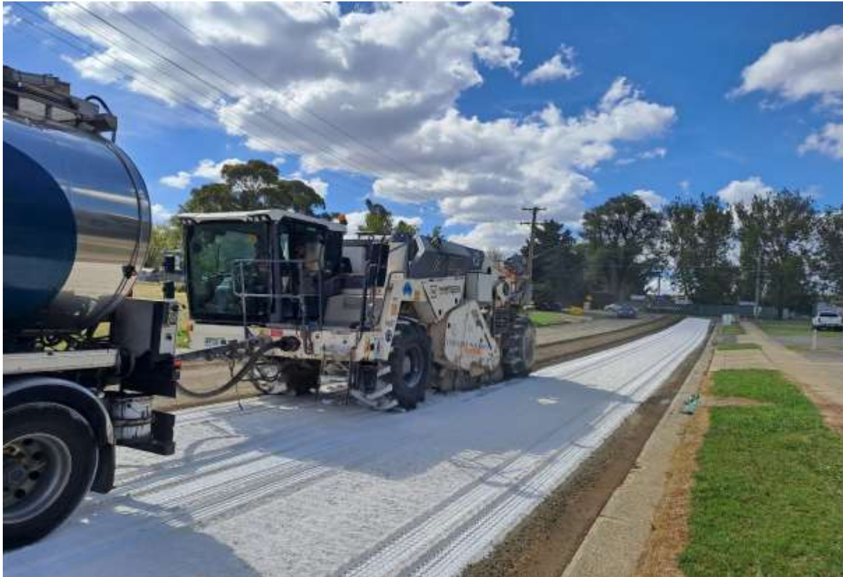
Photo – Road reclaimer connected to hot bitumen tanker, McLachlan Street
