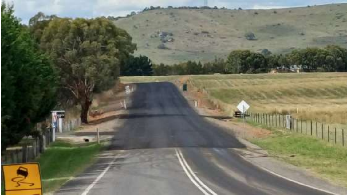
Photo: Seal applied to pavement upgrade between Blunt and Beaumah Road
