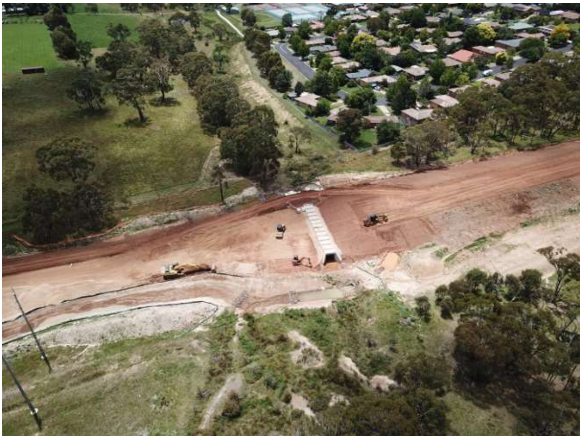
Photo: Culvert Rifle Range Creek
