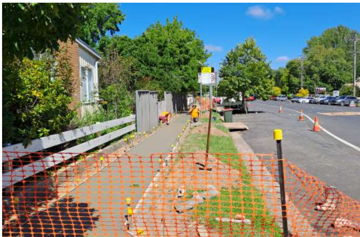
Photo: Footpath reconstruction in Moulder Street
