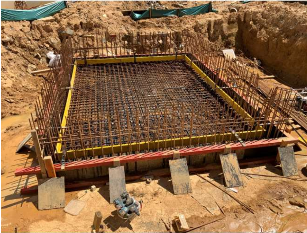
Photo: Preparation for pump station slab pour
