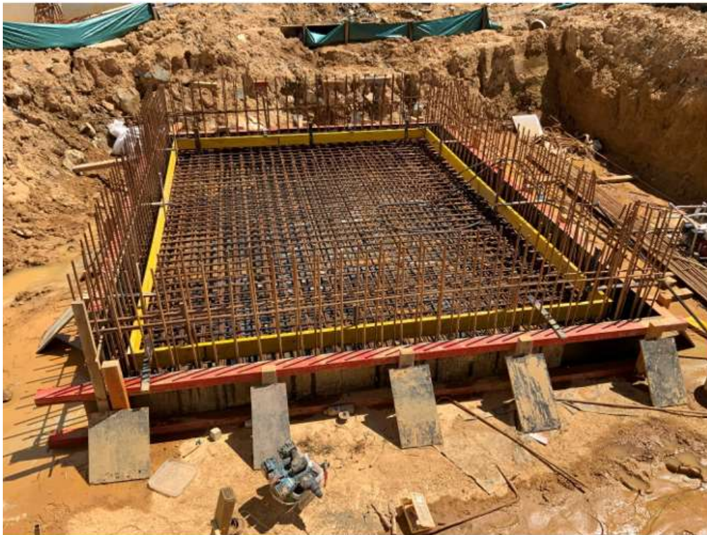
Photo: Preparation for pump station slab pour
