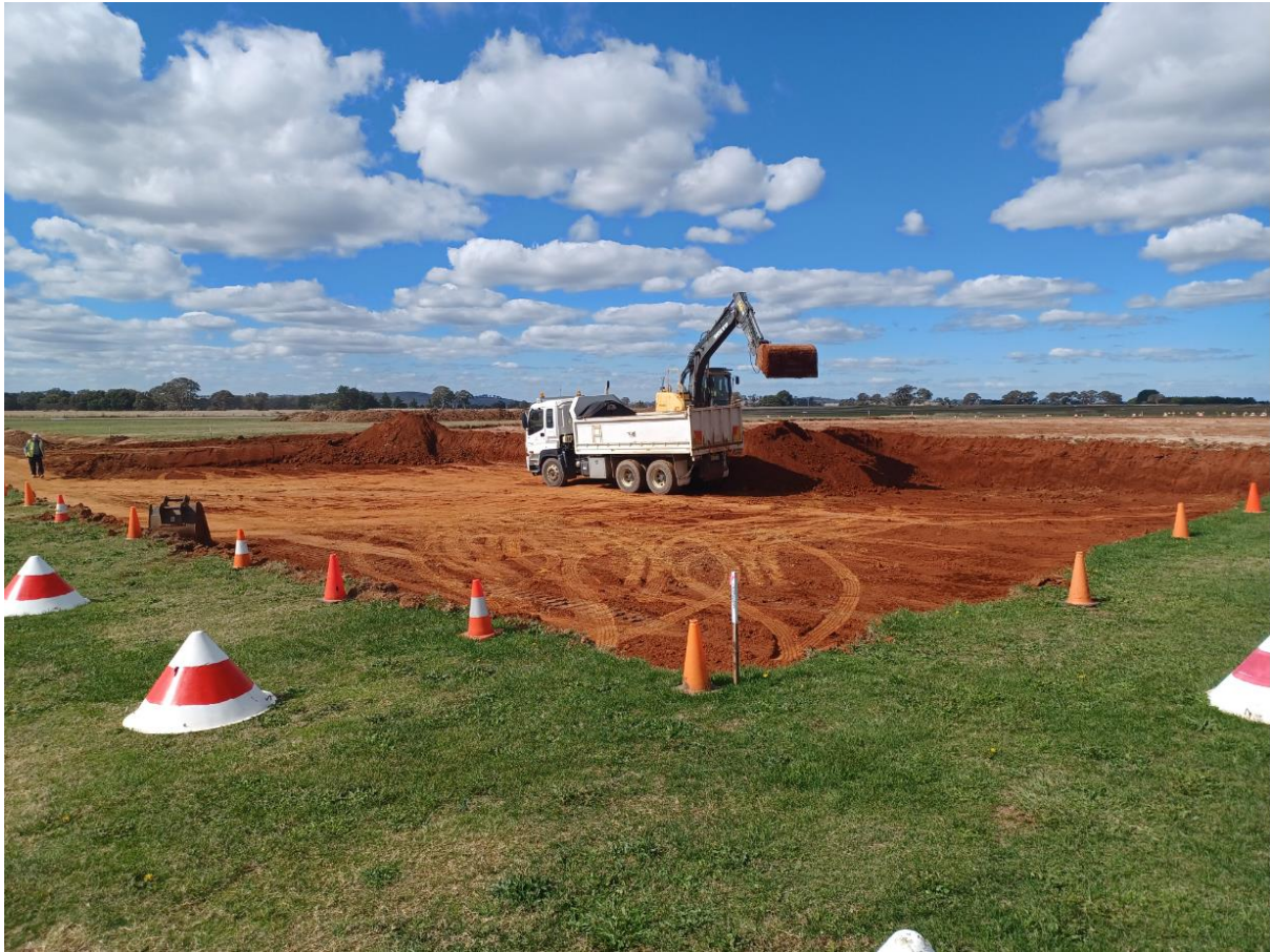
Photo: Excavation for airport hardstand area
