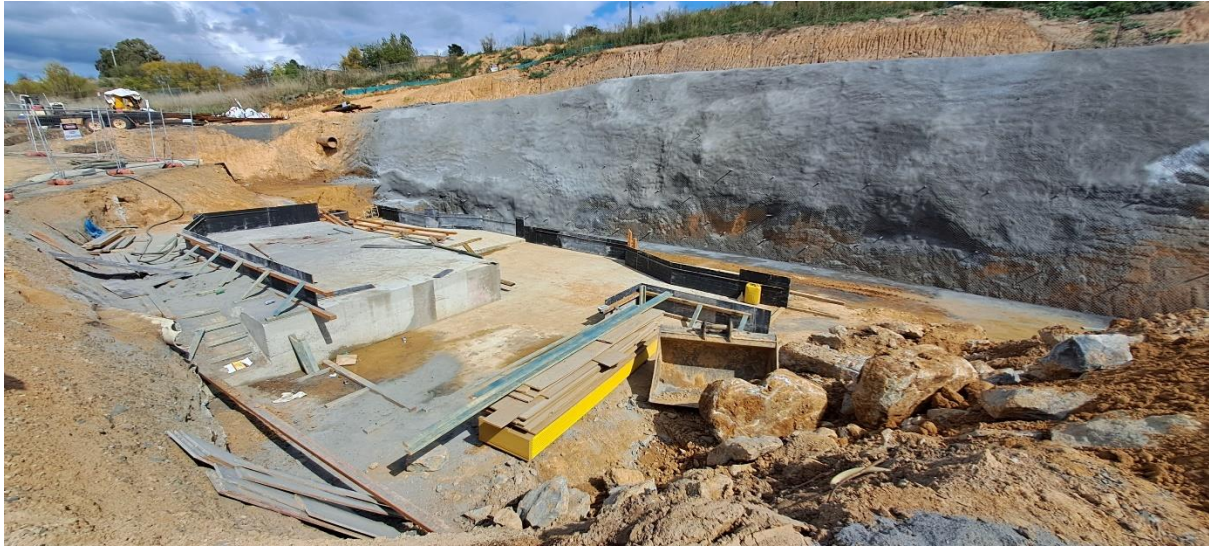
Photo: Sewage Treatment Plant Inlet Works Shotcrete
