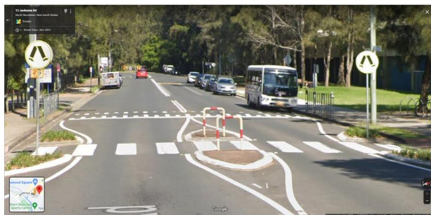
Figure 7 – Pedestrian crossing with refuge, Jacksons Road, North Narrabeen. Refuges are often supplemented with kerb blisters or extensions
