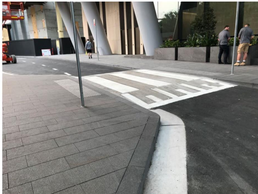
Figure 8 – Raised pedestrian crossing, Parramatta Station, Parramatta. A kerb extension has been installed on one side of the crossing to narrow the width of the crossing and to provide pick-up/drop-off bays close to the station entrance.
