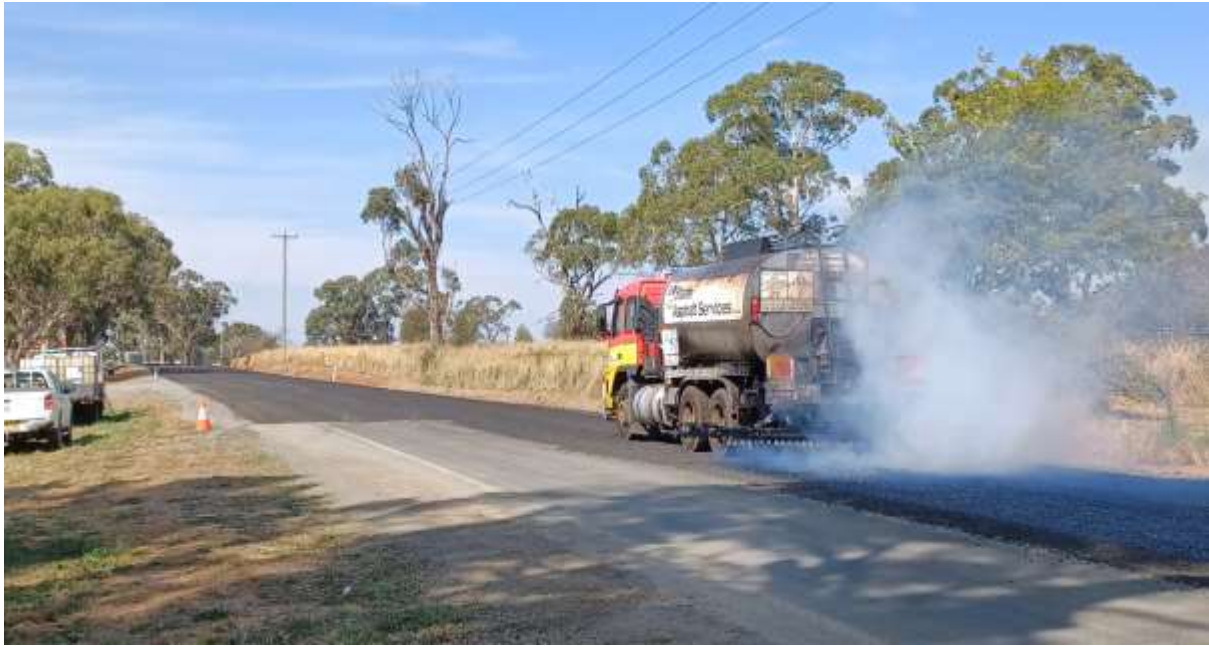
Photo – Sealing new works on Forest Road
