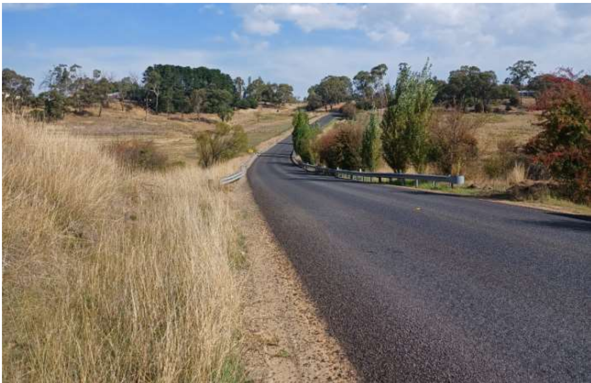
Photo – Recently completed road upgrade of Huntley Road
