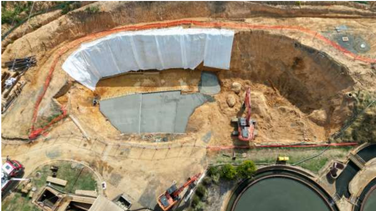
Photo: Sewage Treatment Plant Inlet Works
