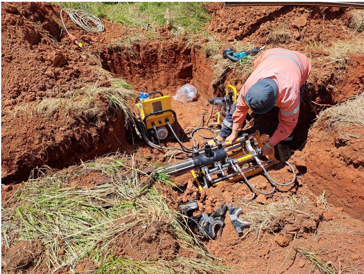
Photo: Butt welding of pipe joints
