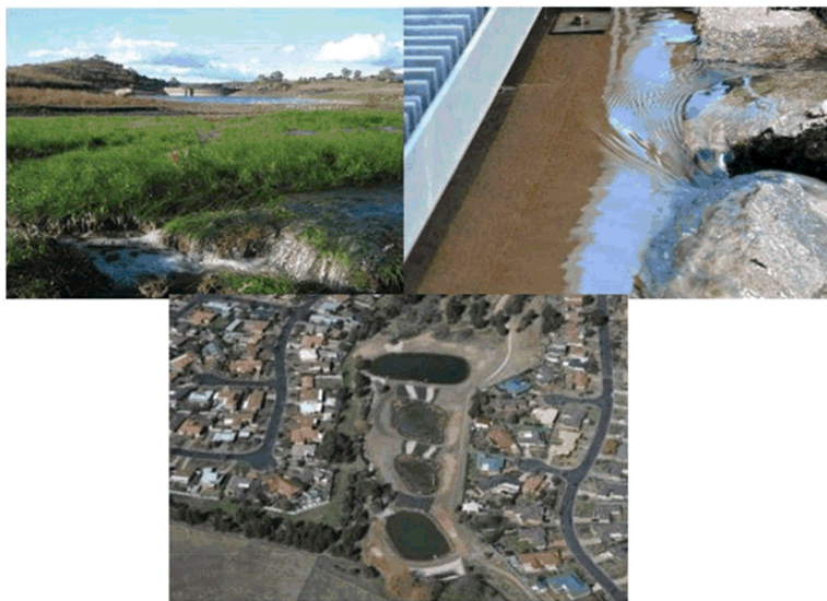
Figure 21 Orange City's stormwater harvesting projects.
