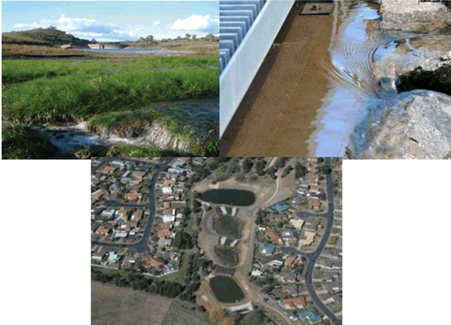
Water and stormwater harvesting in Orange
