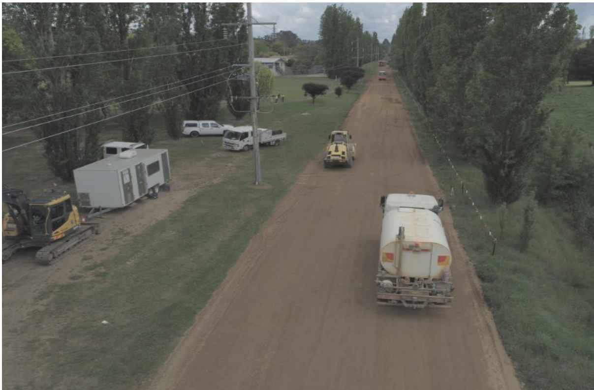
Photo: Rolling of Ploughmans lane following chemical stabilisation
