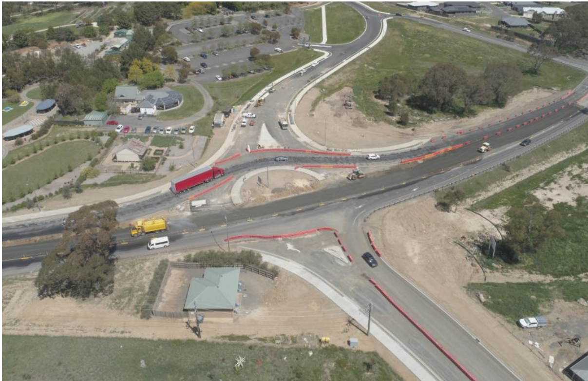
Photo: Traffic switch to new roundabout pavement Westbound
