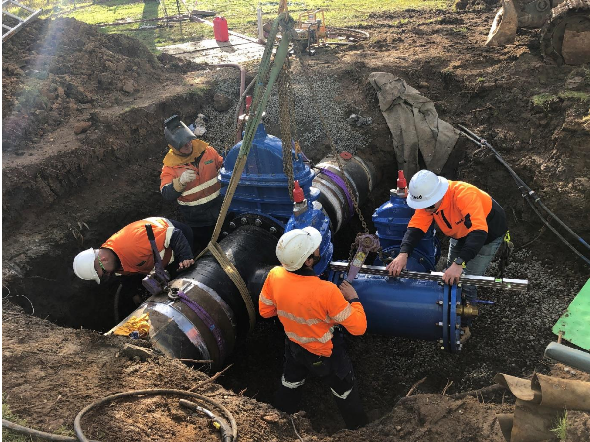
Connection of the pipeline into the 600mm raw water main at the Icely Road Water Treatment Plant
