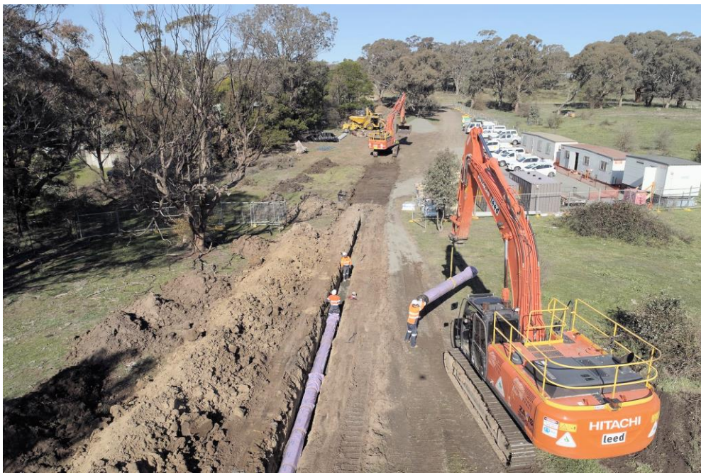
Photo: Leed Engineering installing pipework near their compound approaching Icelly Road
