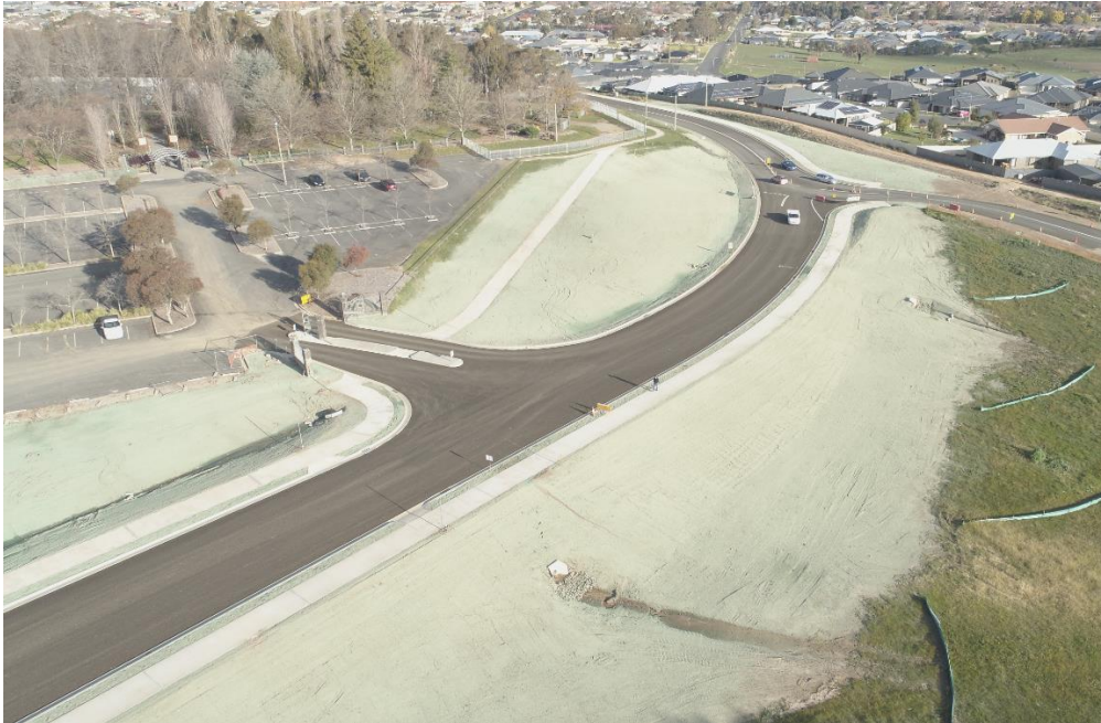
Photo: Seal applied to Hill Street realignment
