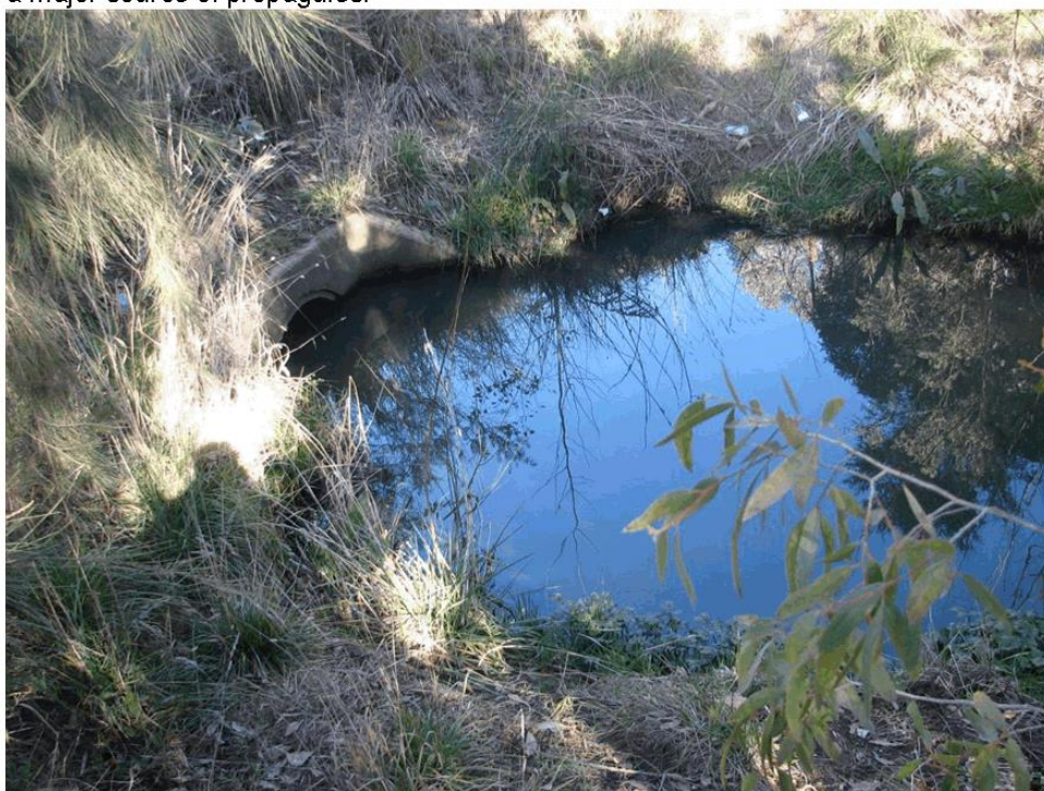
Figure 2.63. Item 2. Immediately downstream of Kearneys Drive. Pipe half drowned, suggesting scouring and deposition downstream. Armouring of the stream base will be needed if a detention basin is built upstream
