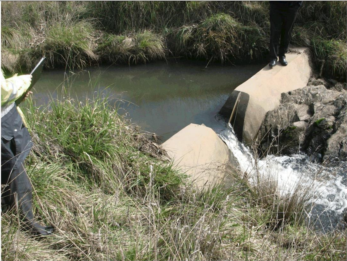
Figure 2.33. The V notch weirs provide an hydraulic jump which can result in a scour pool and undercut banks.
