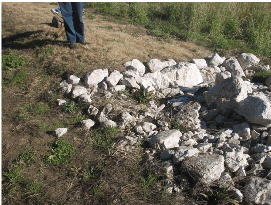
Figure 2.47. Item 5. Rocked batter between ponds 3 and 4. The rocks are being outflanked. The site needs include graded edges to prevent lateral flows and an armoured base to prevent scouring on top of the bank. Rocks with D_{50} of 500 mm are needed. Rabbits are evident.
