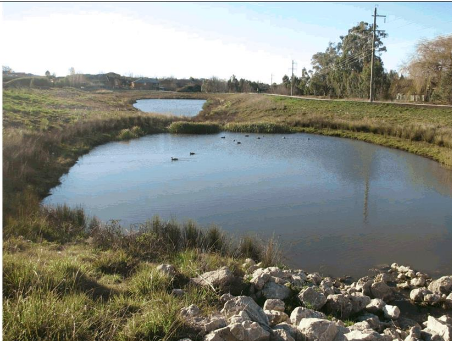
Figure 2.16. Item 4. The fringing vegetation is sparse, and provides little cover for birdlife. Additionally children could readily access the water. Thicken up vegetation see item/site 4 in table 2. Also add clumps of suitable fringing trees. See item/site 5.
