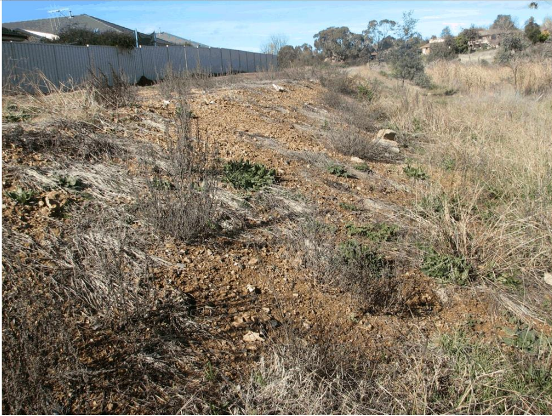
Figure 2.72. The top, face and toe of the building platform runs parallel to the right hand side of the stream line. It needs revegetation.
