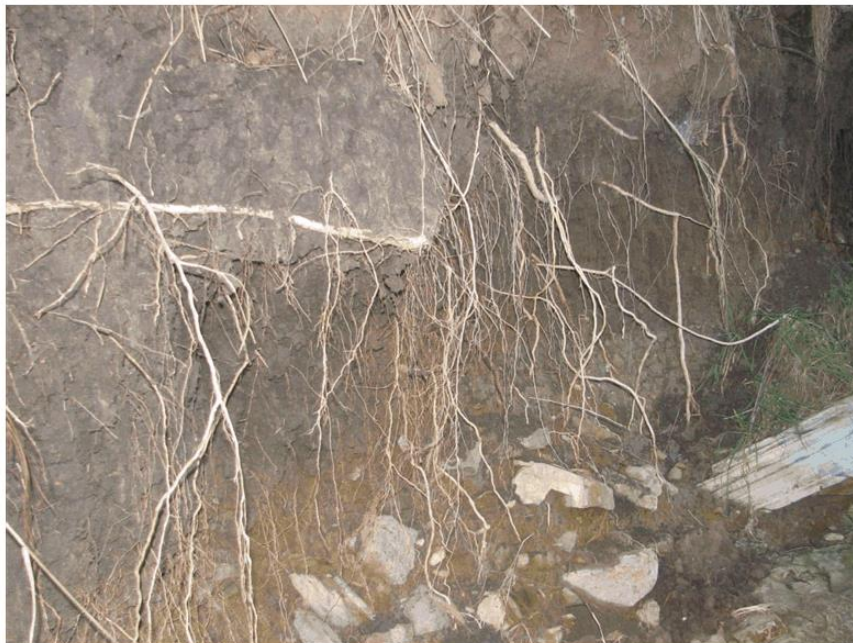
Figure 2.54. Item 2. The waterway is incised over 2m. Plant roots will provide little resistance to erosion at the depth. Laying back the banks would assist, but it is expensive and probably not worthwhile as the length of waterway involved is relatively short.
