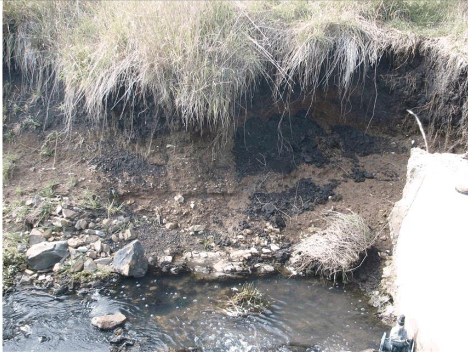
Figure 2. 57. Item 4. The concrete block containing the V notch weir has been outflanked. This has resulted in severe undercutting of the right hand bank. It needs stabilisation. The concrete block needs extending at least 1 m into the bank. The bank needs armouring at this point.
