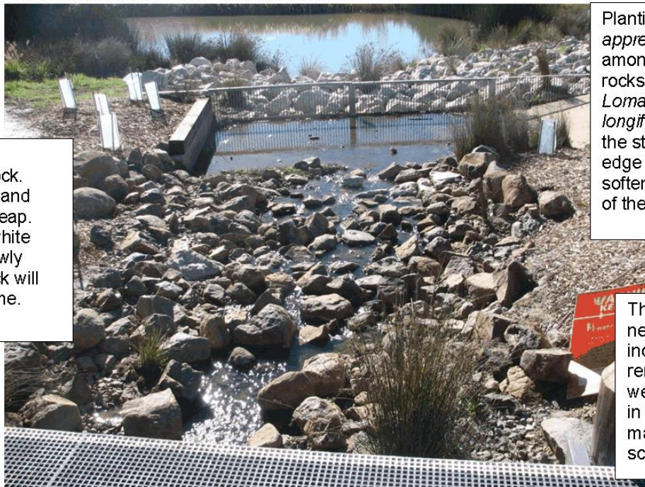
Figure 2.7. Site 4. This trash rack is probably not necessary as the upstream wetland would provide filtering. The rocks upslope of the rack are too small. Conversely the ones downstream protrude above the base of the rack. Replace current small rocks upslope of the rack with rock with a D_{50} of around 400 mm (Engineering Dept may have information on catchment size, imperviousness and anticipated peak flows. This information is needed to determine correct rock size).
