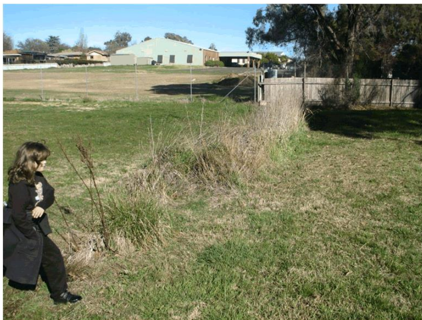
Figure 2.37. Well vegetated swale drains minimise urban impacts on streams. Leave a unmown strip 2m wide on each side of the drain.
