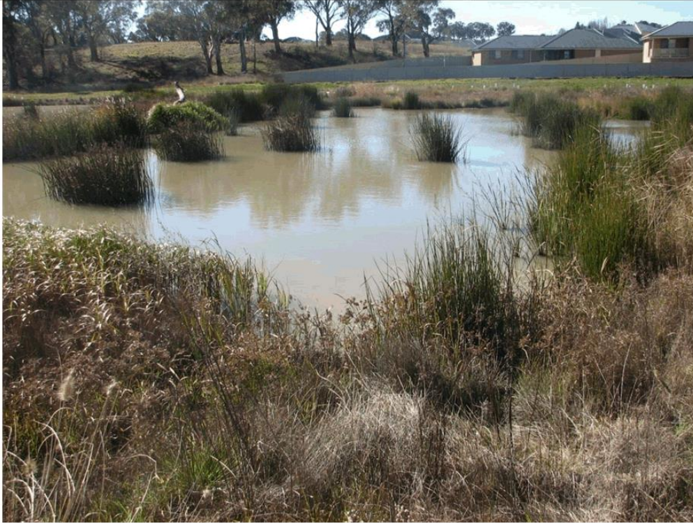
Figure 2.78. Item 4. Water in the Brooklands Wetland is turbid. This is not from upstream as the inflowing water is clear. Erosion and sediment mobilisation from nearby building sites will rapidly fill the wetland. Increasing the buffer width around the wetland to 15m will assist.
