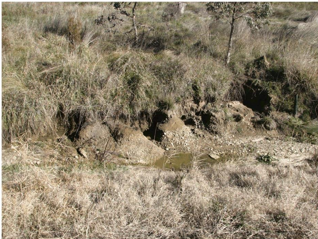
Figure 2.71. Severe channel erosion due to increased flow from Botanica Way.
