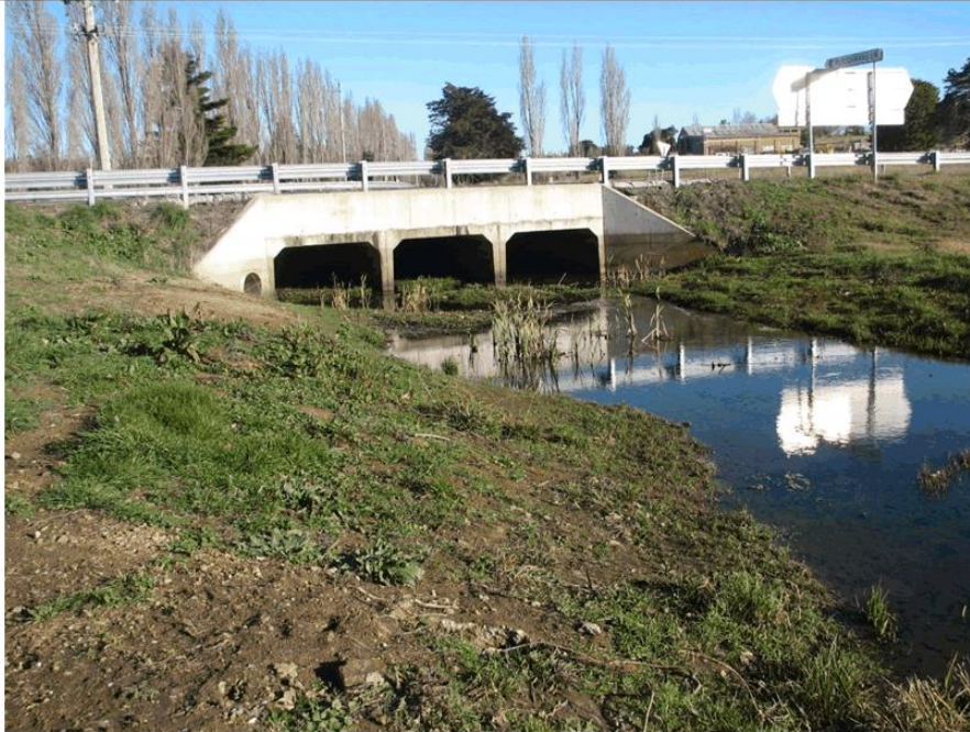
Figure 2.14. Item 1. There are significant quantities of road base entering the wetlands. Erosion management along the roads could be better. (It will become a significant issue during housing development. Alternatively consider installing a vault covered with a 50*50mm mesh. This would need to be capable of being cleaned out with an excavator bucket.
