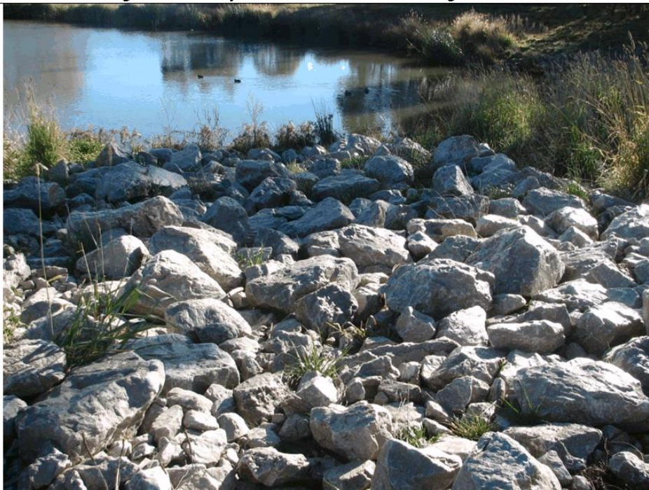
Figure 2.46. Item 4. Entry to lowest pond. Rocks are too small and are therefore moving.
