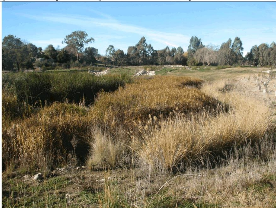
Figure 2.44. Item 2. The fringing aquatic plant zone is especially wide in this wetland cell. This is probably because it has a shallow grade in the pond. The thick vegetation reduces the risk of children accessing it. A 15m wide unmown buffer is required.
