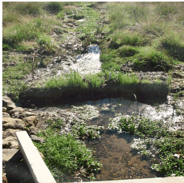
Figure 2.5. Site 2. There is no energy dissipater at this site (see appendix A for design criteria). The hay bales are outflanked by high flows. Sediment, including road base, is an issue.
