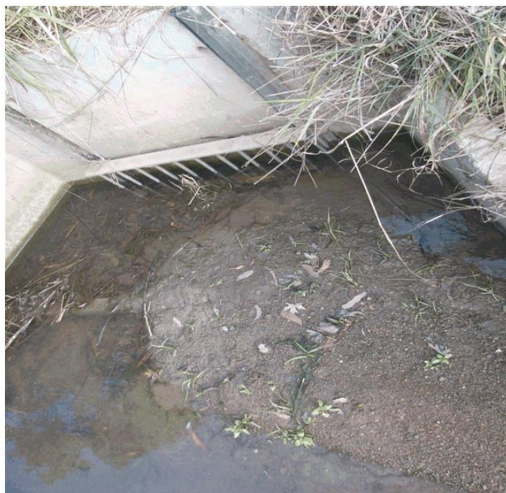
Figure 56. Item 3. The water harvesting off take is partly blocked with sediment. Sediment accumulation in the pump-well will be extremely difficult to clean out.
