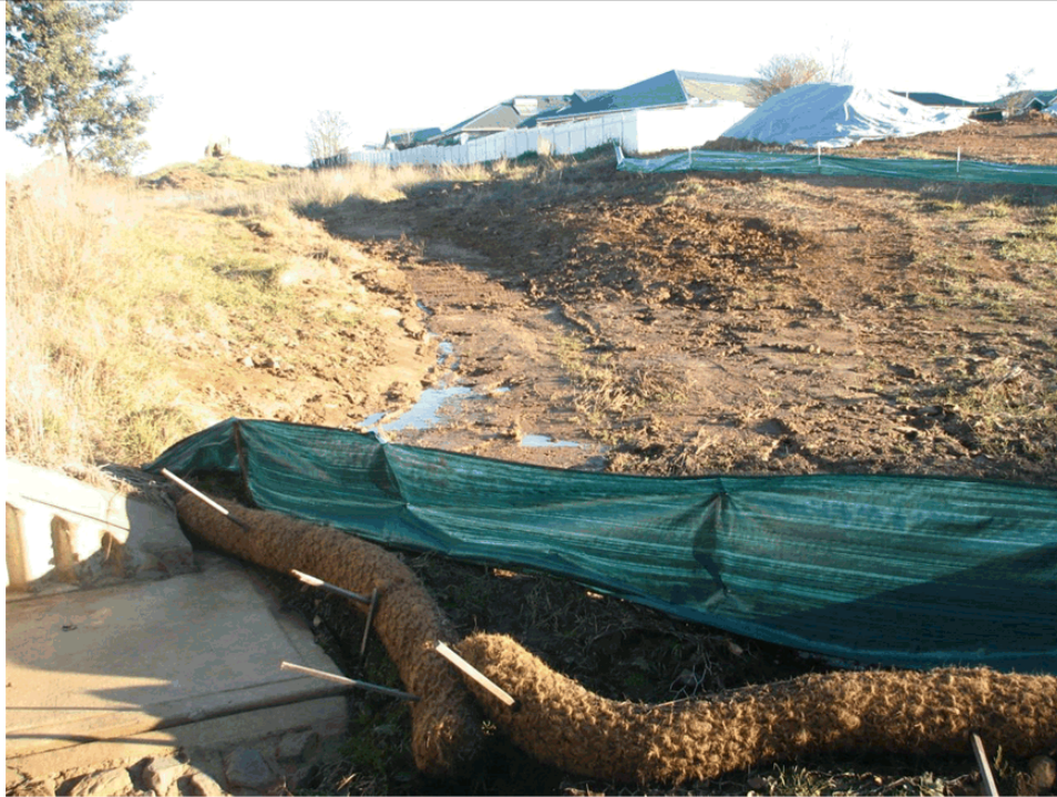
Figure 2.21 Item 9. Poor erosion and sediment control increases sediment influx to wetlands. The silt fence is sitting above the ground surface. The coir logs have 'rolled' and are ineffectual.
