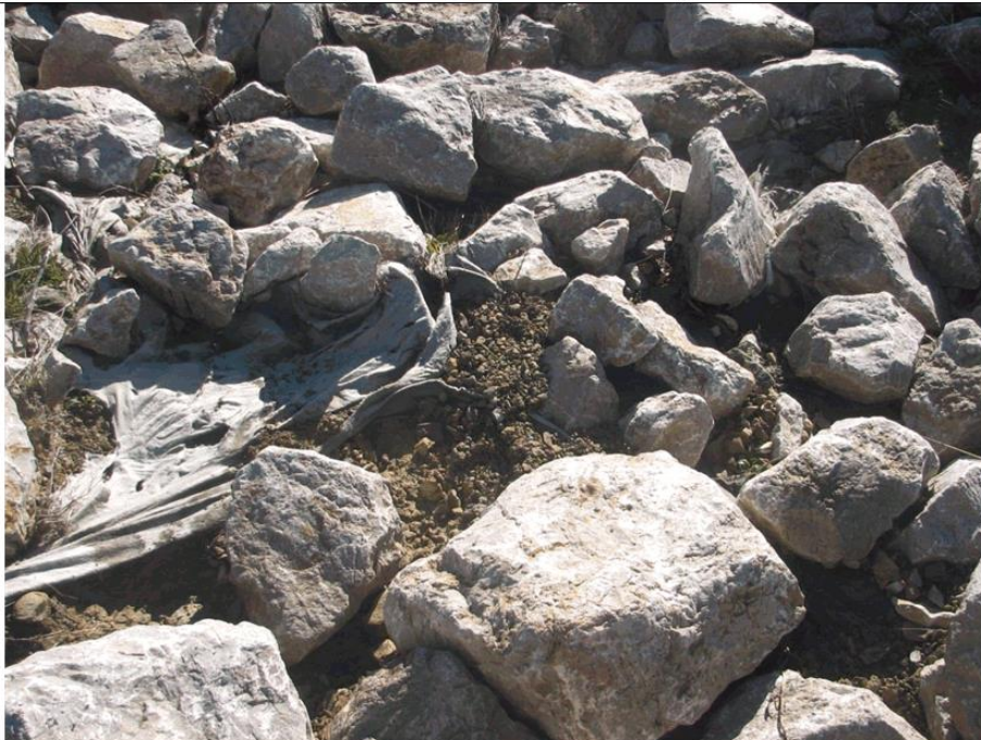
Figure 2.48. Item 6. The geofabric has been damaged and there is extensive deposition of coarse sediment among the rocks.
