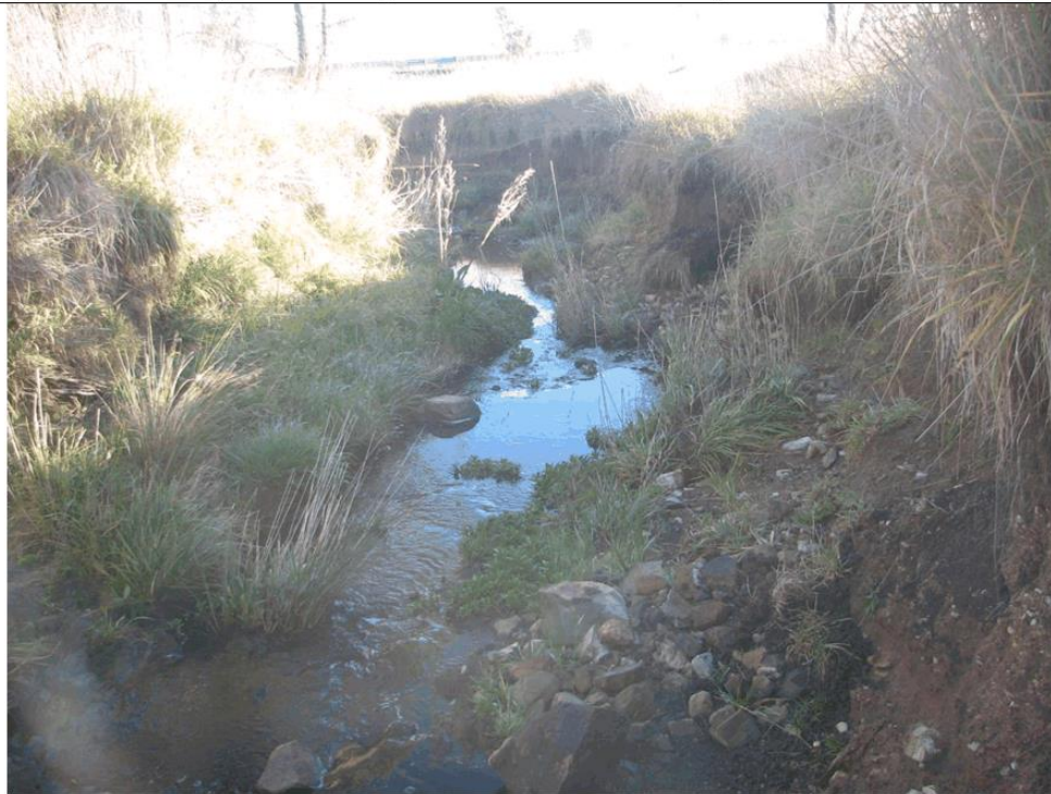
Figure 2.59. Item 2. The reach below the V notch weir is deeply incised. The near vertical banks are unstable. The ideal treatment would be to 'lay' the banks back to 2.5 to 3 : 1 H:V, then plant out with full suite of riparian vegetation. However this would be an expensive operation.
