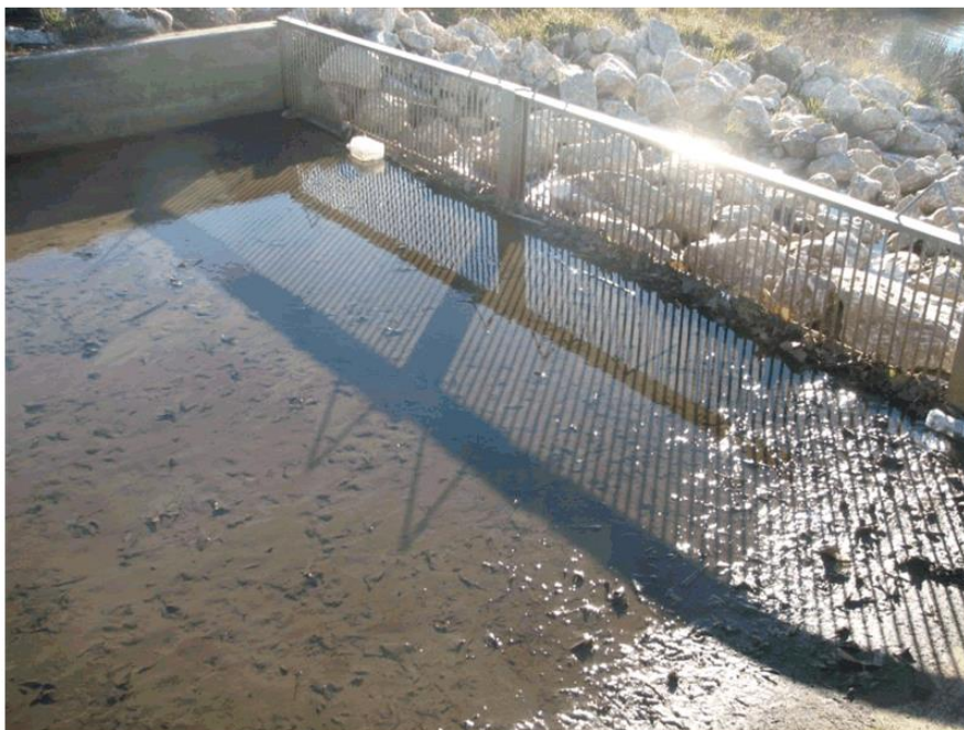
Figure 2.15. The trash rack has minimal ability to capture sediment because there is no plinth at the base. Additionally there is no 'return at the top so PET bottles can float away. The rocks below the rack are too small given the catchment size (and therefore the likely peak flows). Additionally the rocks protrude above the concrete basin. There is significant influx of road base.
