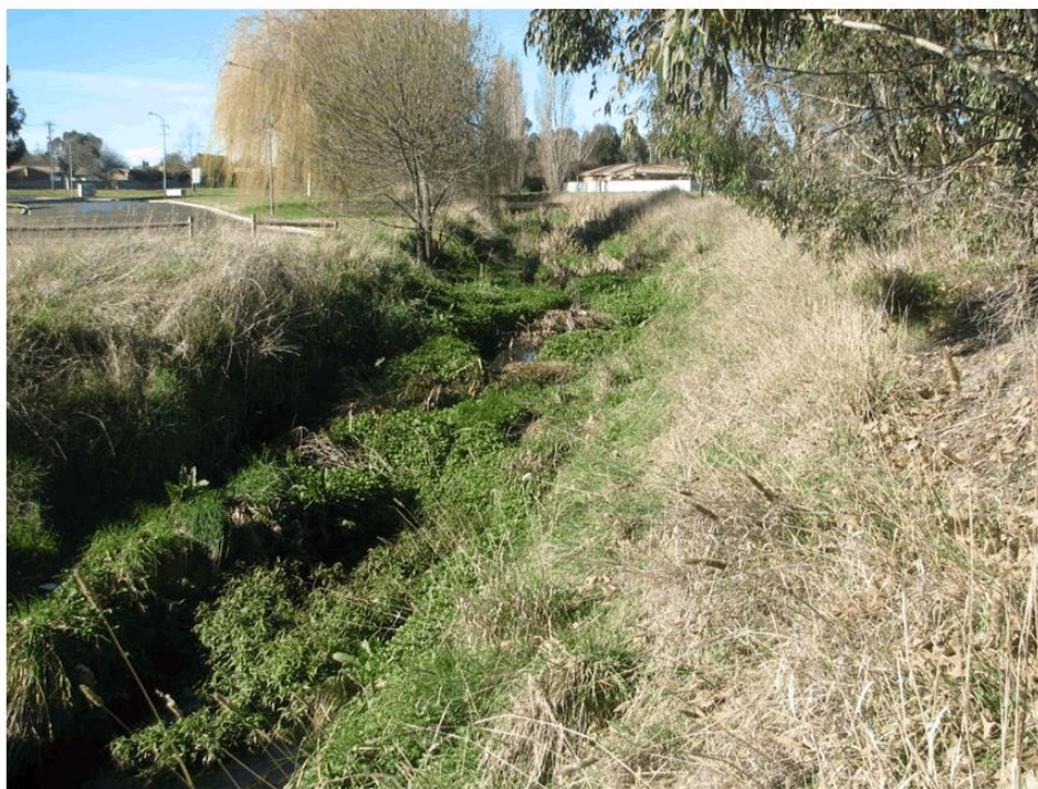
Figure 2.36. The Somerset Park Tributary is incised near the top end of its catchment. However the banks are well vegetated. Removal of willows and addition of euclypts and other native plants would assist stabilisation.
