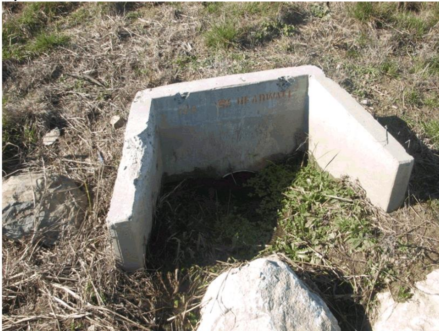
Figure 2.79. Inflow pipes are becoming blocked.
