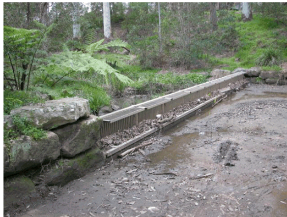
Figure A2.1. This trash rack design allow for retention of sediment and debris at the base. It also has a return which facilitates retention of floating debris when the entire structure is submerged.
