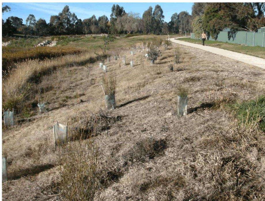
Figure 2.45. Item 3. The 'no-mow' area should extend at least 15m from the top water level in the wetland cells
