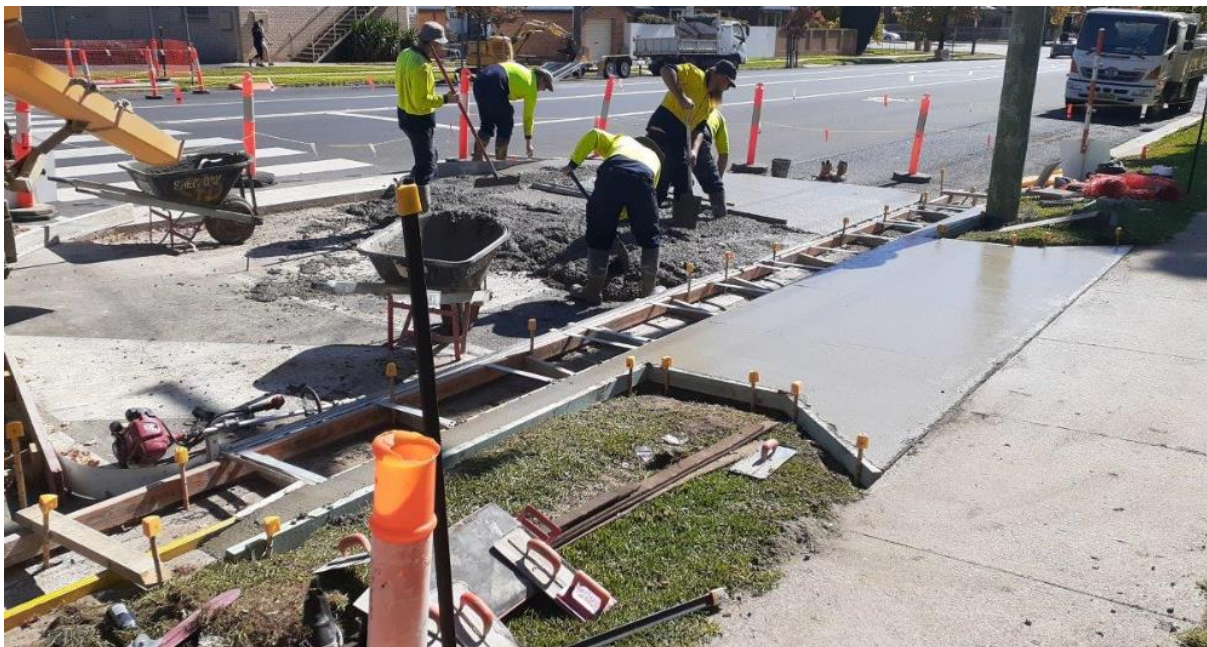
Photo: Concrete pour on eastern side of OPS pedestrian crossing – Anson Street
