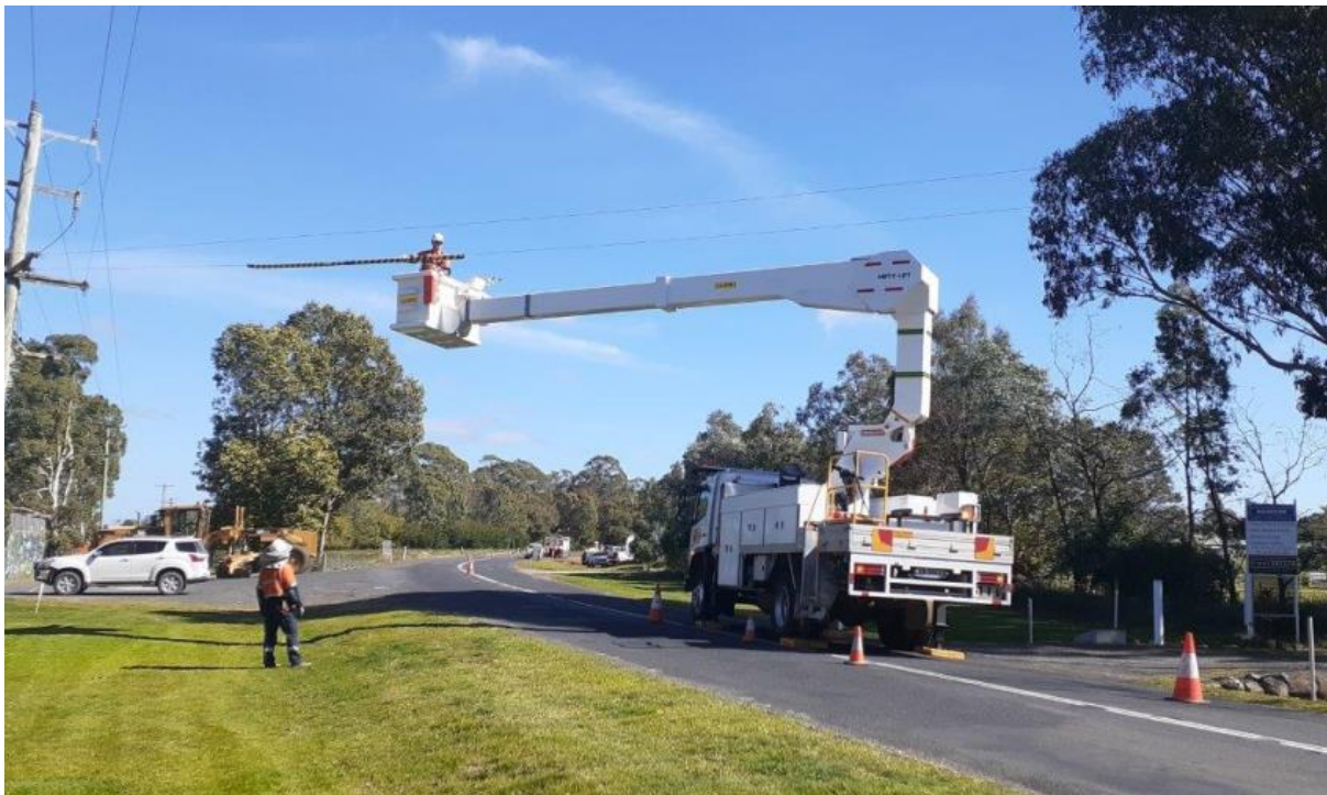
Photo: Essential Energy staff on Forest Road tensioning overhead power lines to achieve maximum road clearance and providing warning sleeves (tiger tails) prior to road reconstruction works.
