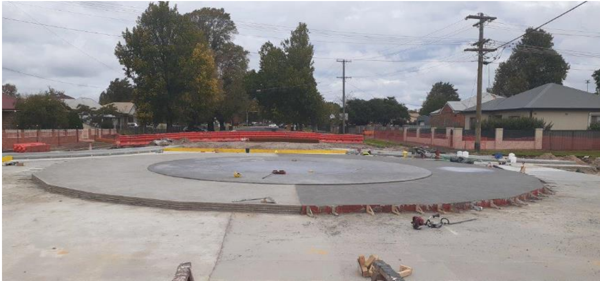
Photo – March and McLachlan: Mountable centre island and first ring of final road pavement
