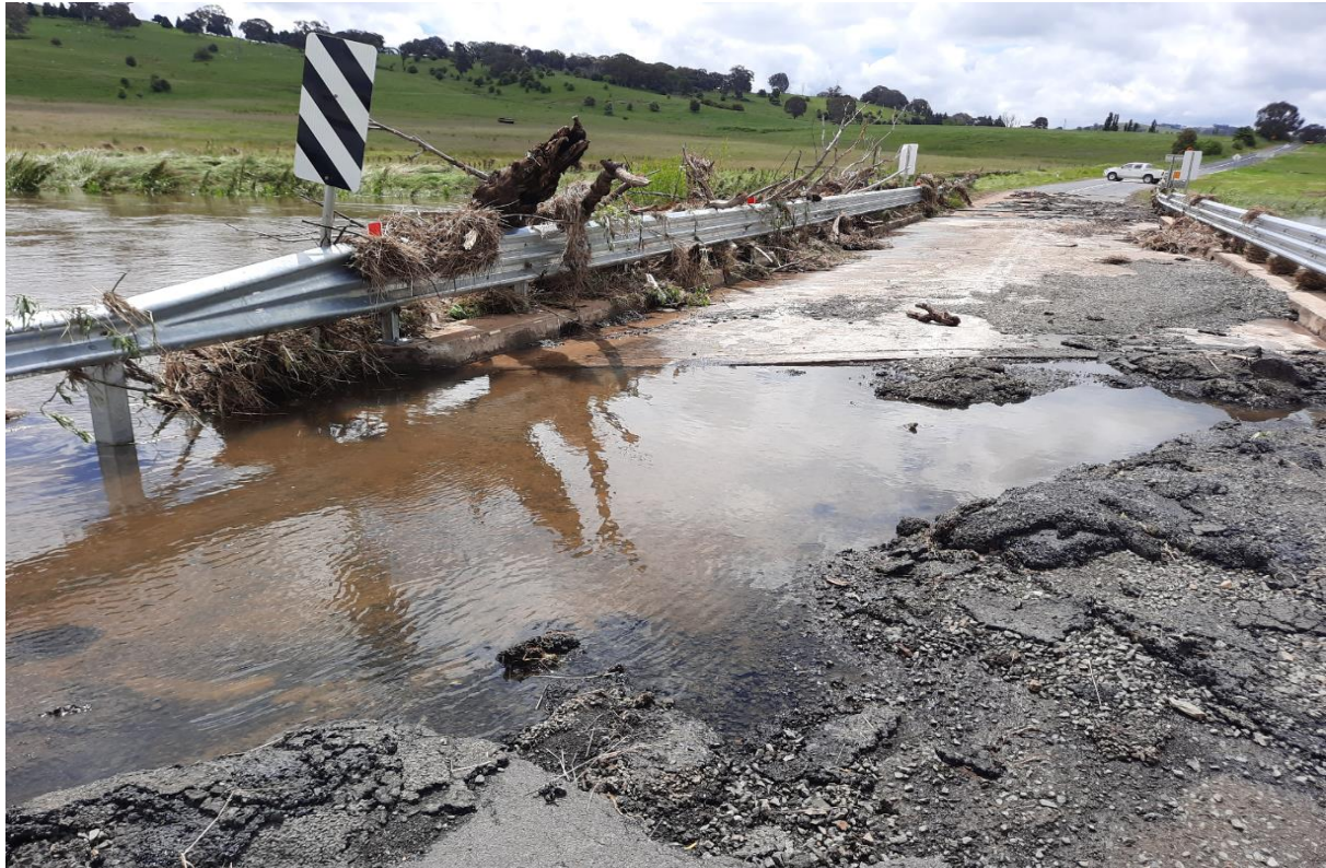
Photo: Debris against bridge and pavement damage at Ophir Road second crossing
