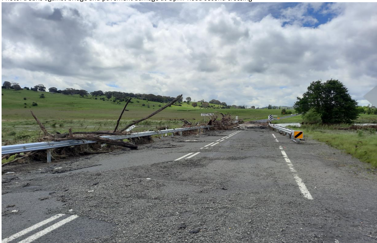
Photo: Debris against bridge and pavement damage at Ophir Road second crossing
