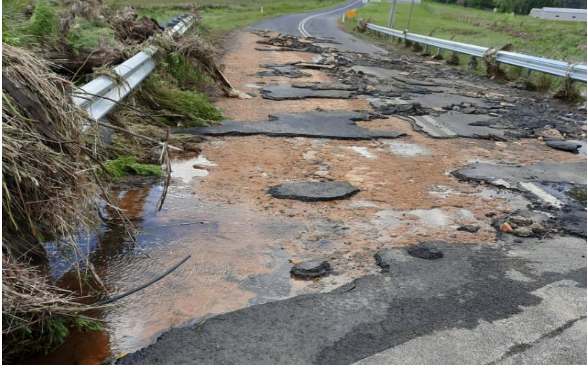
Photos: Debris against bridge and pavement damage at Ophir Road second crossing
