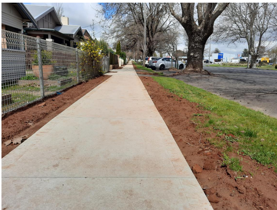
Photo: Footpath re-construction on McLachlan Street
