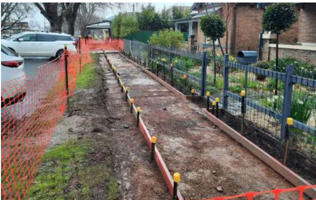
Photo – preparations for the replacement of damaged paths in McLachlan Street
