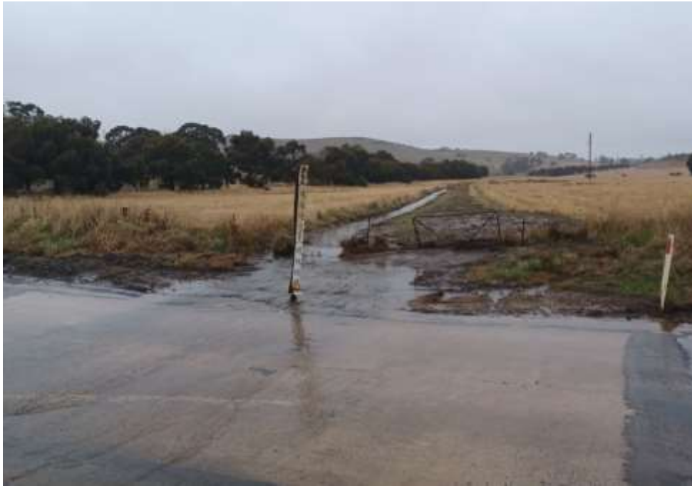
Photo - Clearing of drain through paddock on Beasley Road
